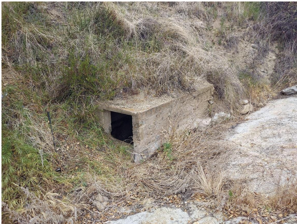
Opening to concrete cistern on downstream side. View to the northeast.
