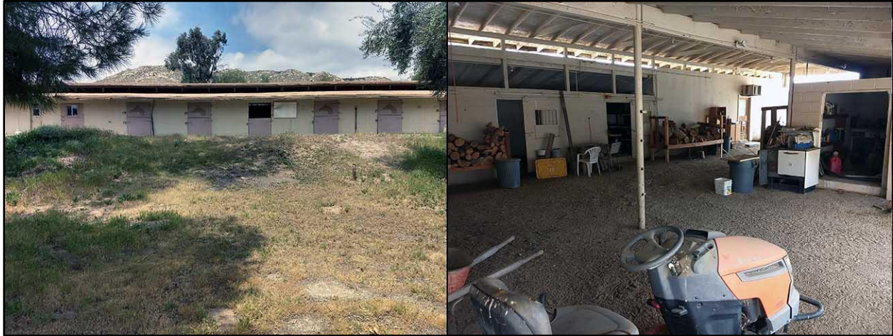
Side stables on the barn and the barn's interior.
