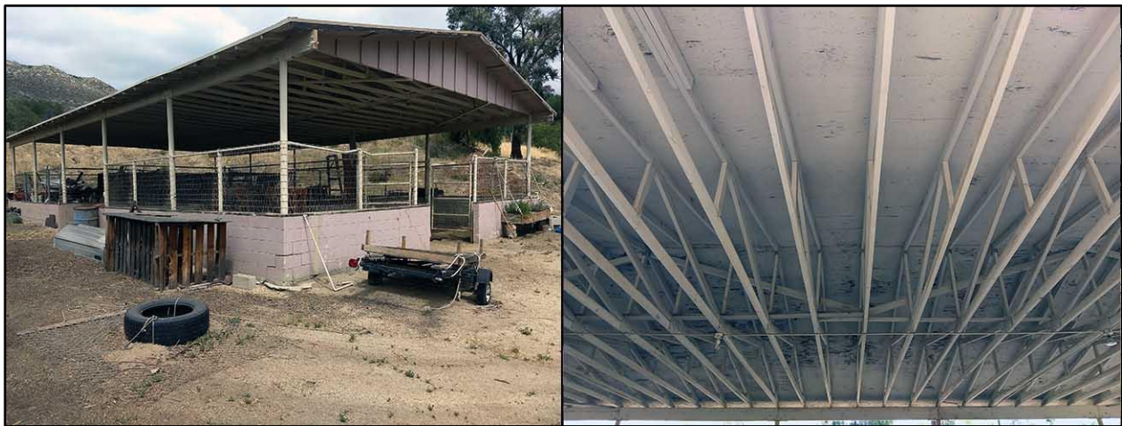
Pole barn (view to the northeast, left) and the barn's rafters.
