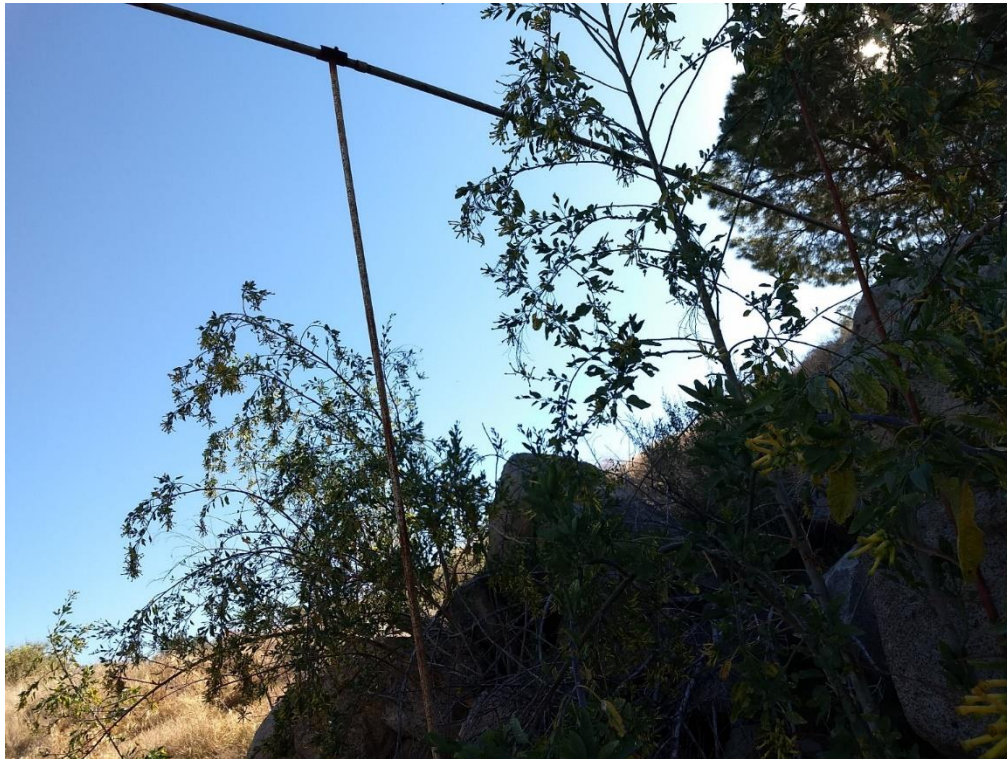
Pipeline entering into slope near levee (Feature 2) View to the northeast.
