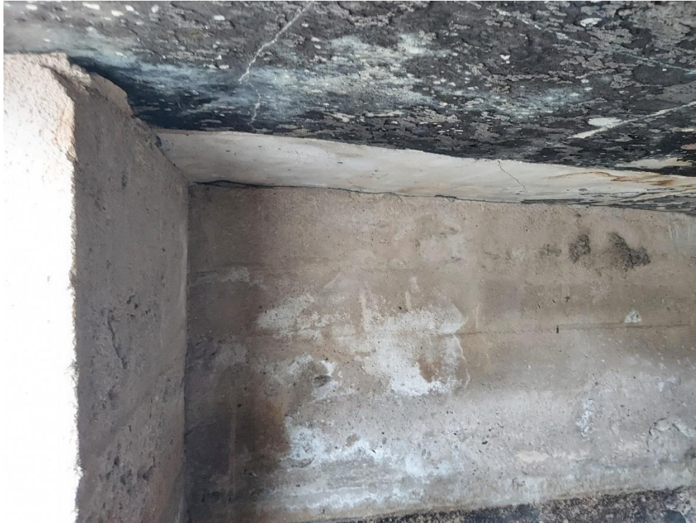
Concrete cistern inside northern wall. View to the north
