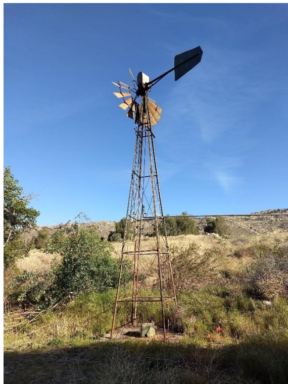
Closeup of windmill. View to the north.
