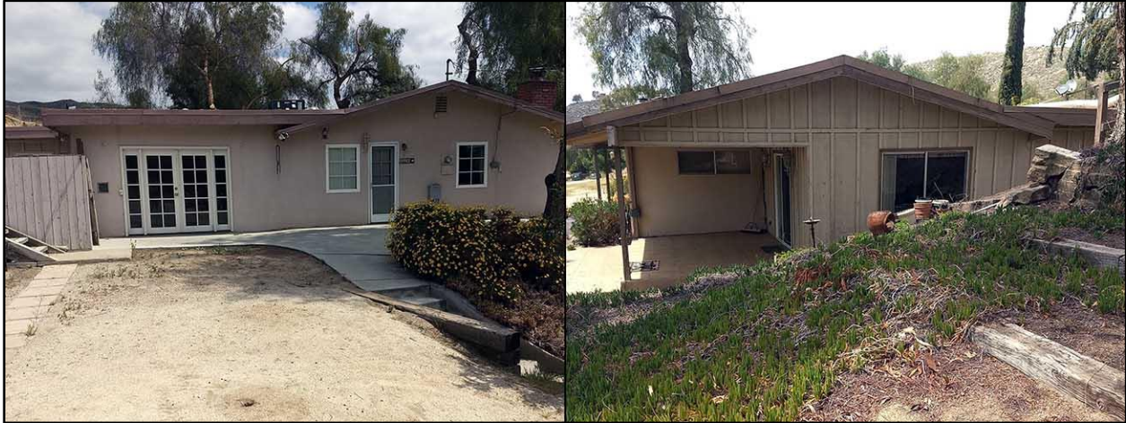
Side views of the residence (to the east, left; to the west, right)
