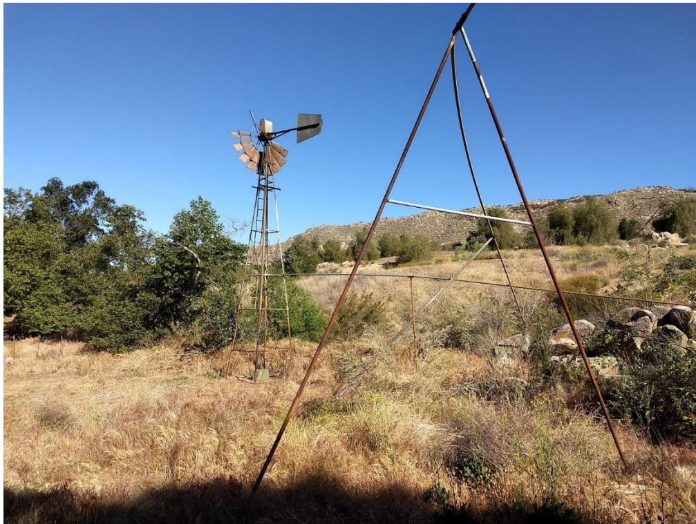
Overview of windmill (Feature 4) and piping structure. View to the northwest.
