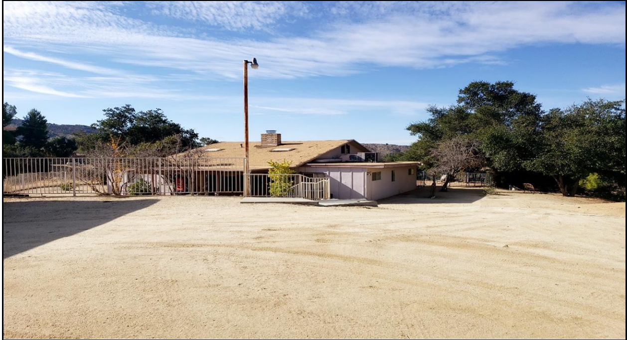
Chaparral House, view to the northwest. (Source: Earth Strata Inc., Dec.2020)
