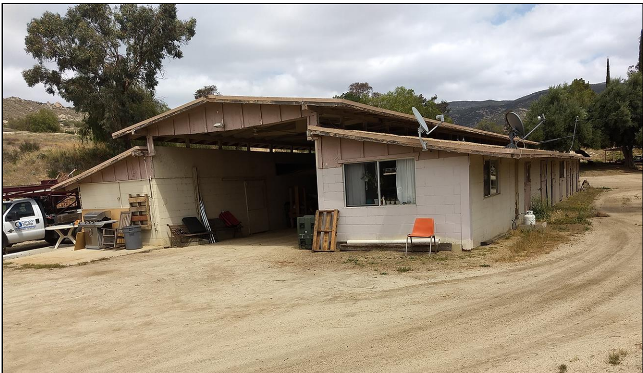
Barn and stables (view to the southwest)
