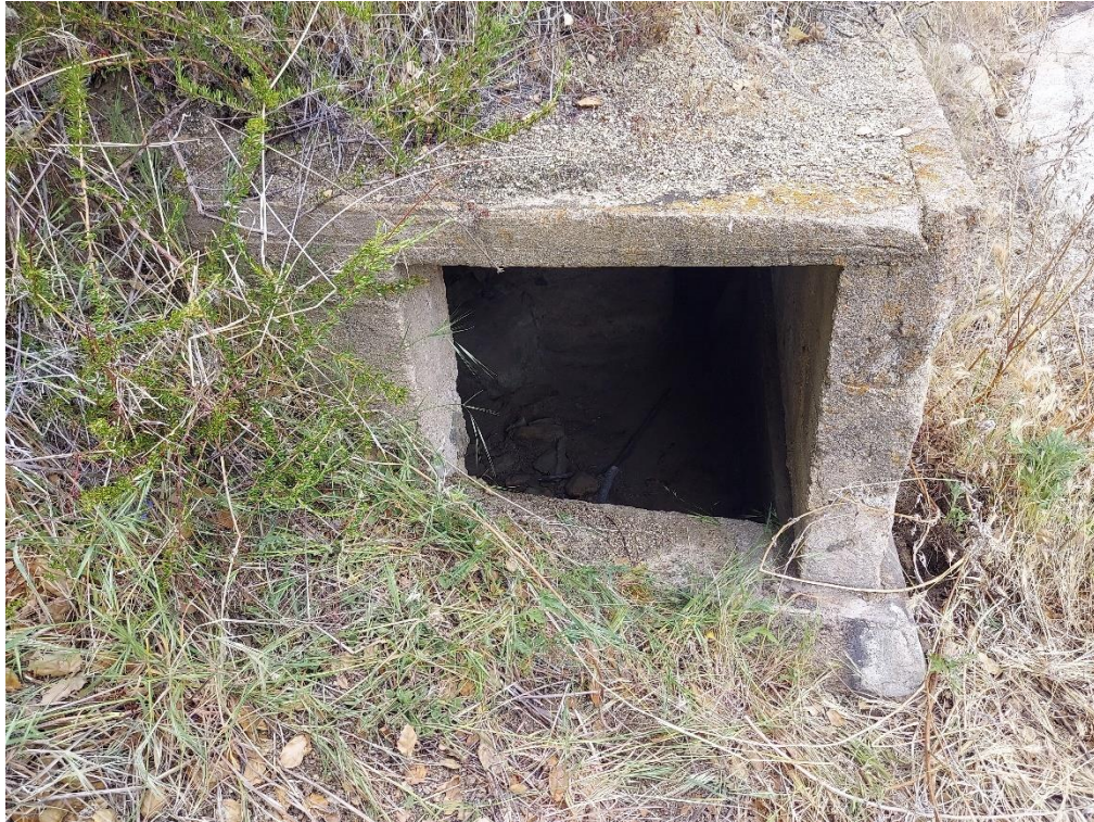
Opening to concrete cistern. View to the east.
