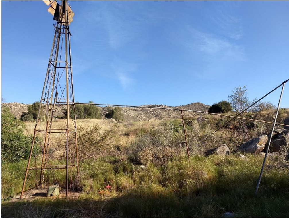
Windmill and pipe structure. View to the north.
