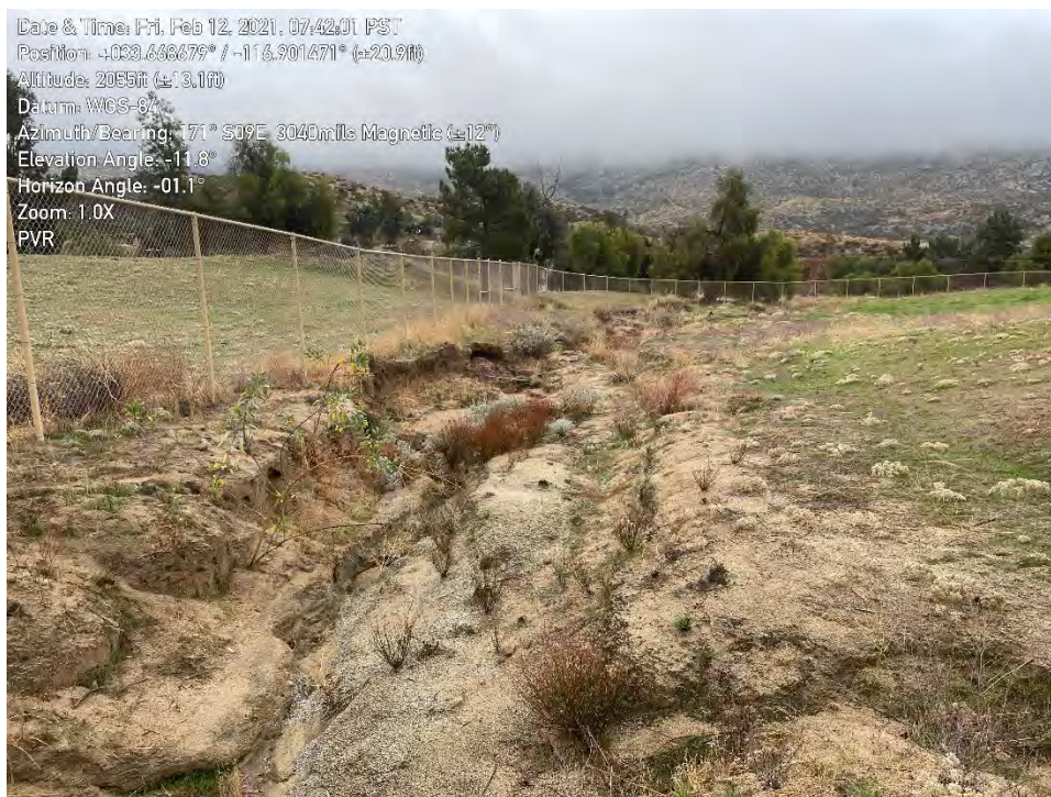
PHOTOGRAPH 12: Feature A 3 downstream of the concrete V-ditch.
