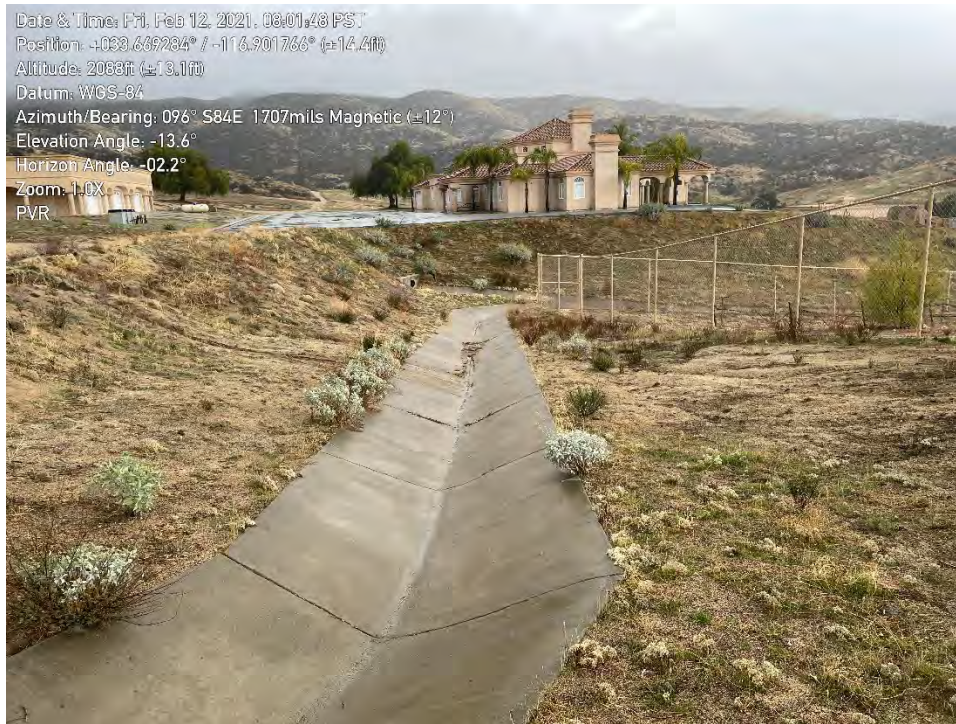
PHOTOGRAPH 11: The concrete V-ditch of Feature A 3 .
