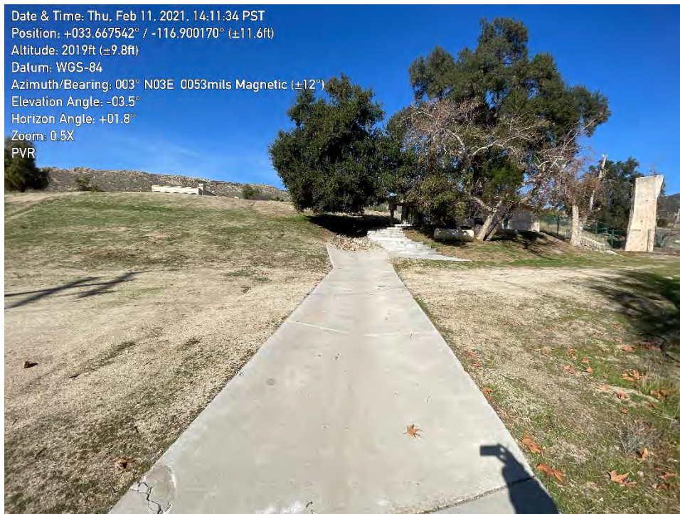
PHOTOGRAPH 10: A concrete apron collecting discharge from the culverts of Feature A 2 .
