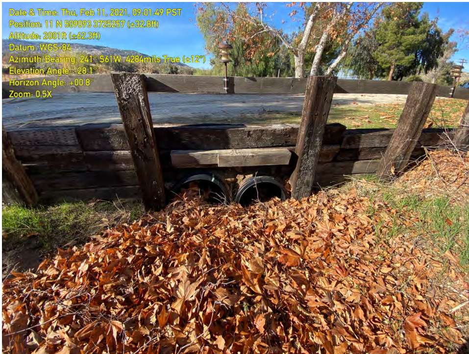
PHOTOGRAPH 2: Two culverts within Feature A located at a dirt road crossing.
