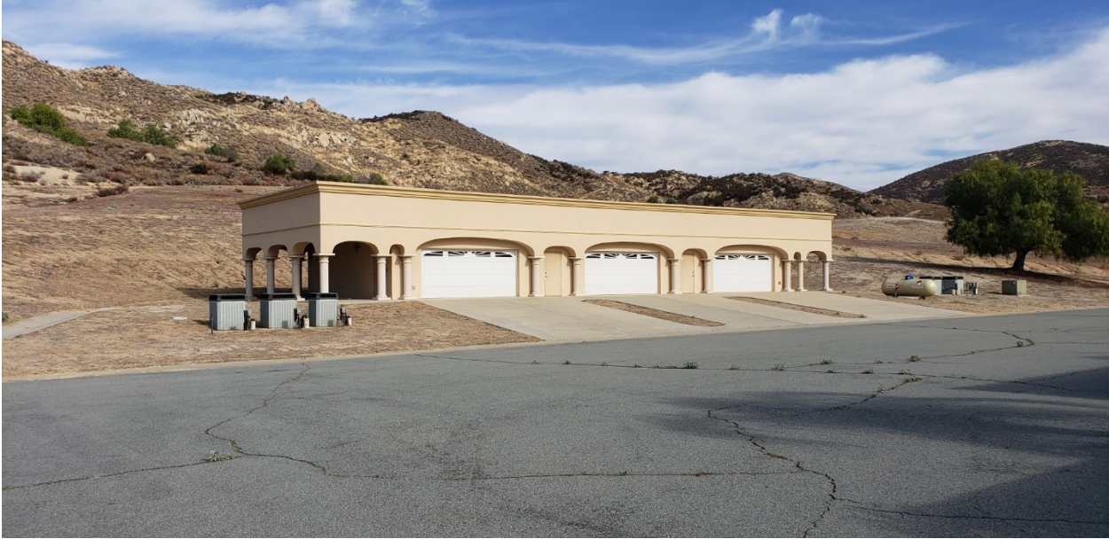
View of garages behind main house looking north. APN 569-020-026
