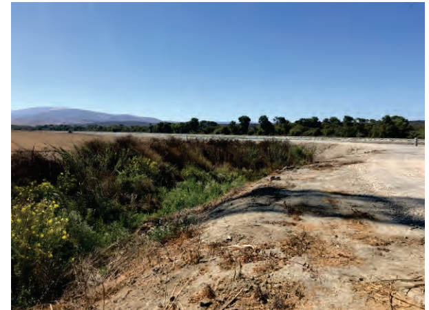
Photo 6. View of the irrigation canal and culvert # 1, facing south. August 11, 2022
