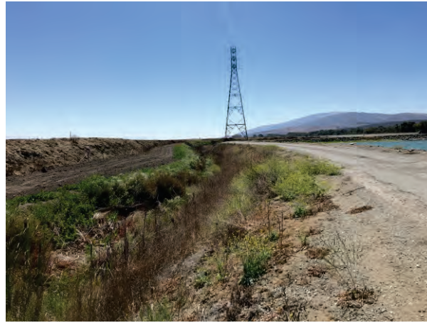
Photo 8. View of the irrigation canal, facing southeast. August 11, 2022
