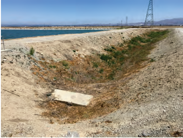
Photo 19. View of the irrigation canal and culvert #4, facing northeast. August 11, 2022
