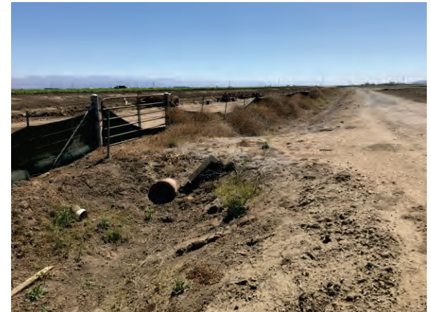
Photo 12. View of culvert #2 and irrigation canal, facing southeast. August 11, 2022
