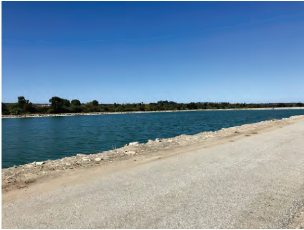
Photo 7. View of the wastewater treatment pond, facing northwest. August 11, 2022
