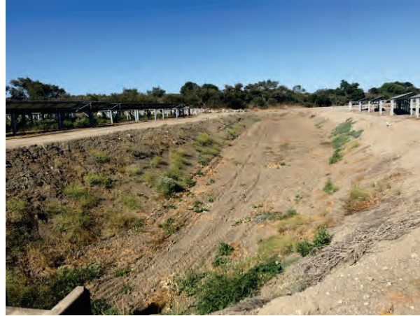
Photo 2. View of the detention basin, facing southwest. August 11, 2022
