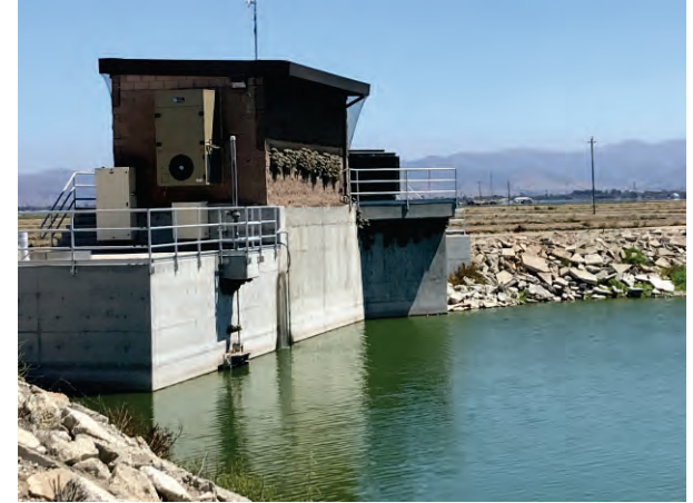
Photo 15. View of the pump house and cliff swallow mud nests, facing northeast. August 11, 2022
