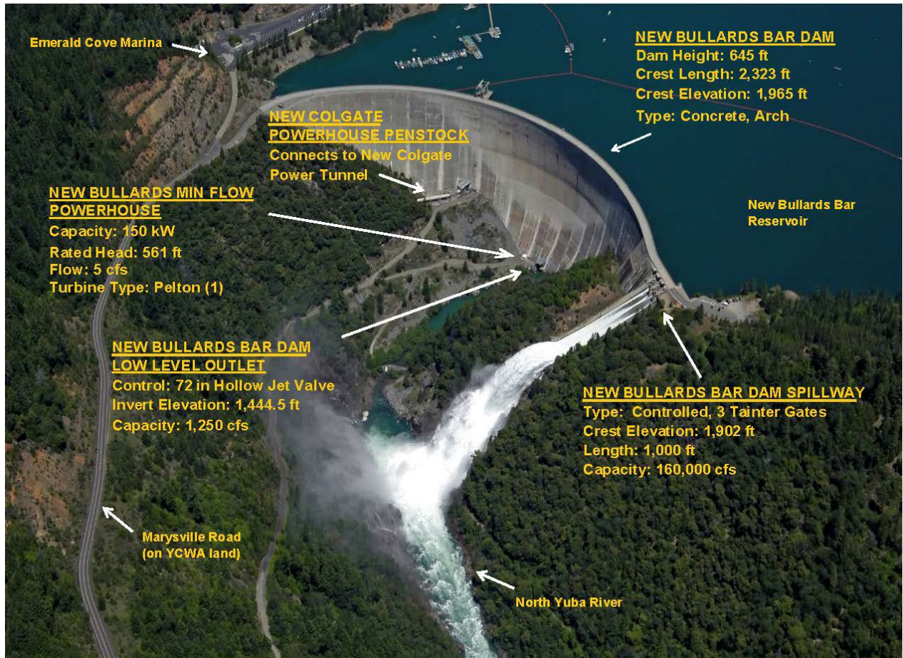
Figure 4-3. New Bullards Bar Dam and associated features.
