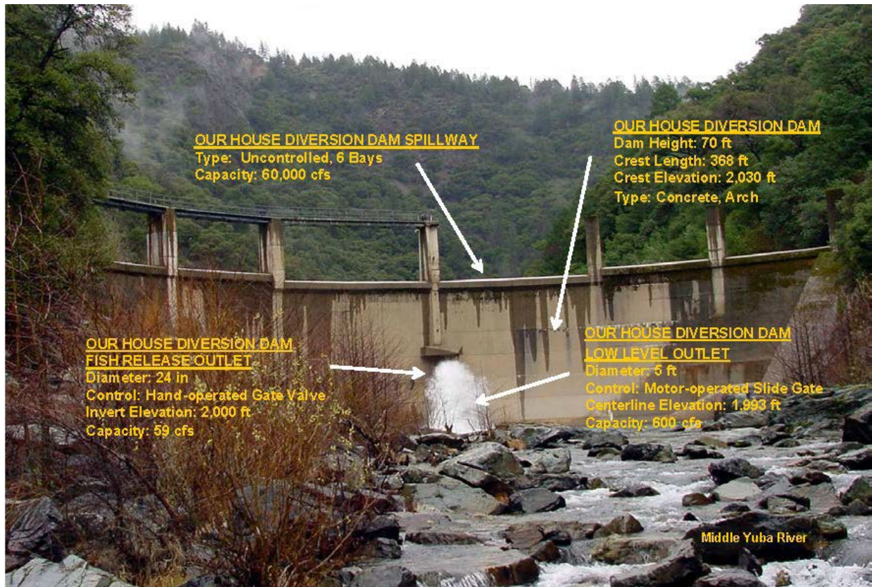
Figure 4-1. Our House Diversion Dam and associated features.
