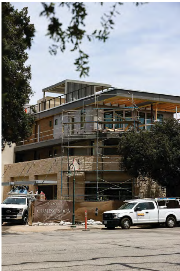
TOP OF THE CITY—Construction is nearing completion at 299 E. Thousand Oaks Blvd. The mixed-use development features 142 units, 11 of which have been designated as “affordable” and will be leased for significantly less than the 131 market-rate apartments. MICHAEL COONS Acorn Newspapers
