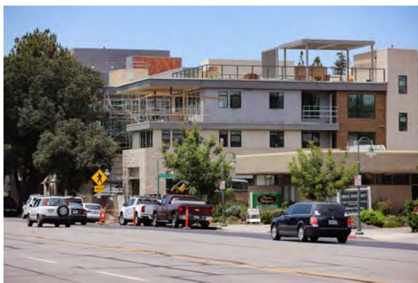
The luxury apartment complex rises above E. Thousand Oaks Boulevard across from Tarantula Hill Brewing Company. Residents are expected to begin moving in sometime in October. Two restaurants, Go Fish Sushi and JOi Cafe, have already signed on to fill the commercial spaces on the bottom floor facing. MICHAEL COONS/Acorn Newspapers
