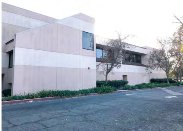
CHANGING HANDS—Amgen’s former Building No. 34 has been sold to the Latigo Group, the same firm developing 299 E. Thousand Oaks Blvd. Last year, Amgen received pre-approval from the council for a concept involving a mix of around 333 apartments and retail on the ground floor. Acorn file photo
