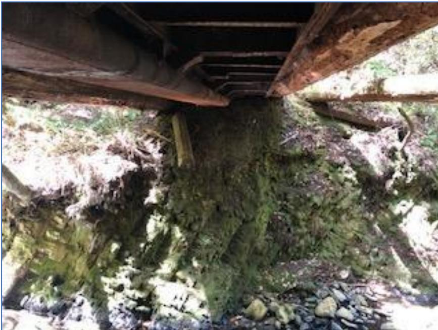
**View 4.** View of underside of existing bridge, showing old railroad car understructure.
