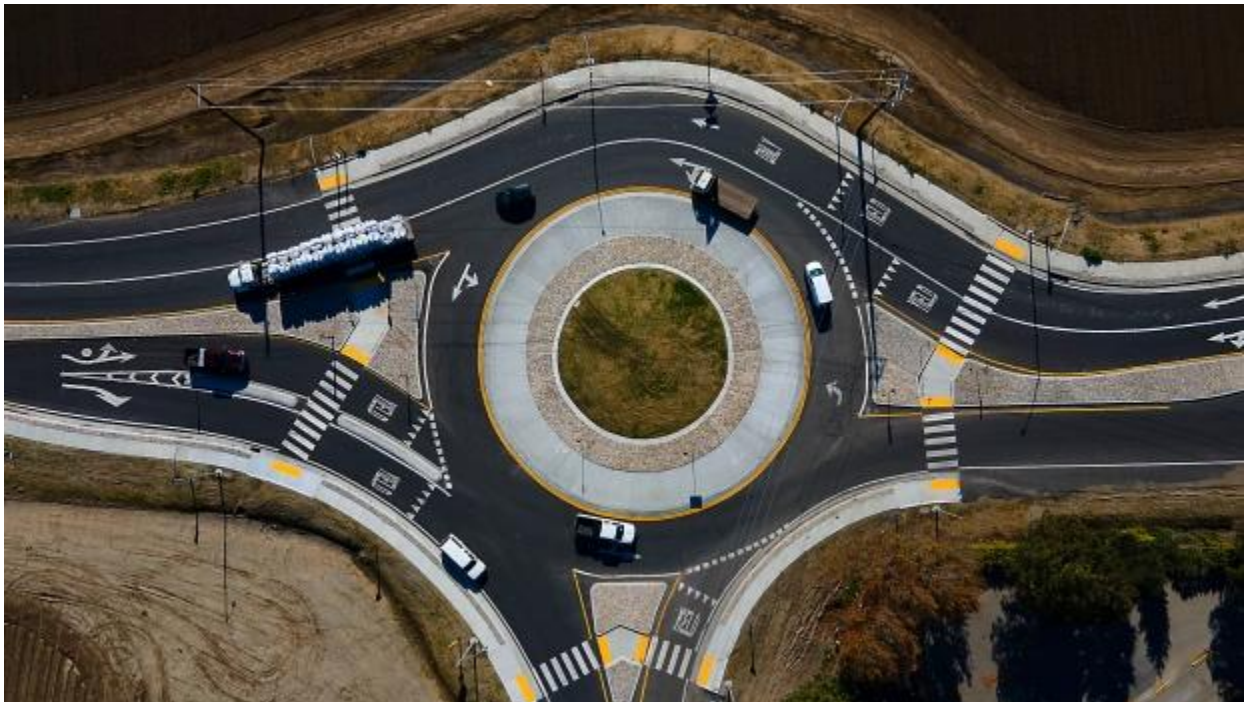
Figure 12: Roundabout at the State Route 129 and Lakeview Road
