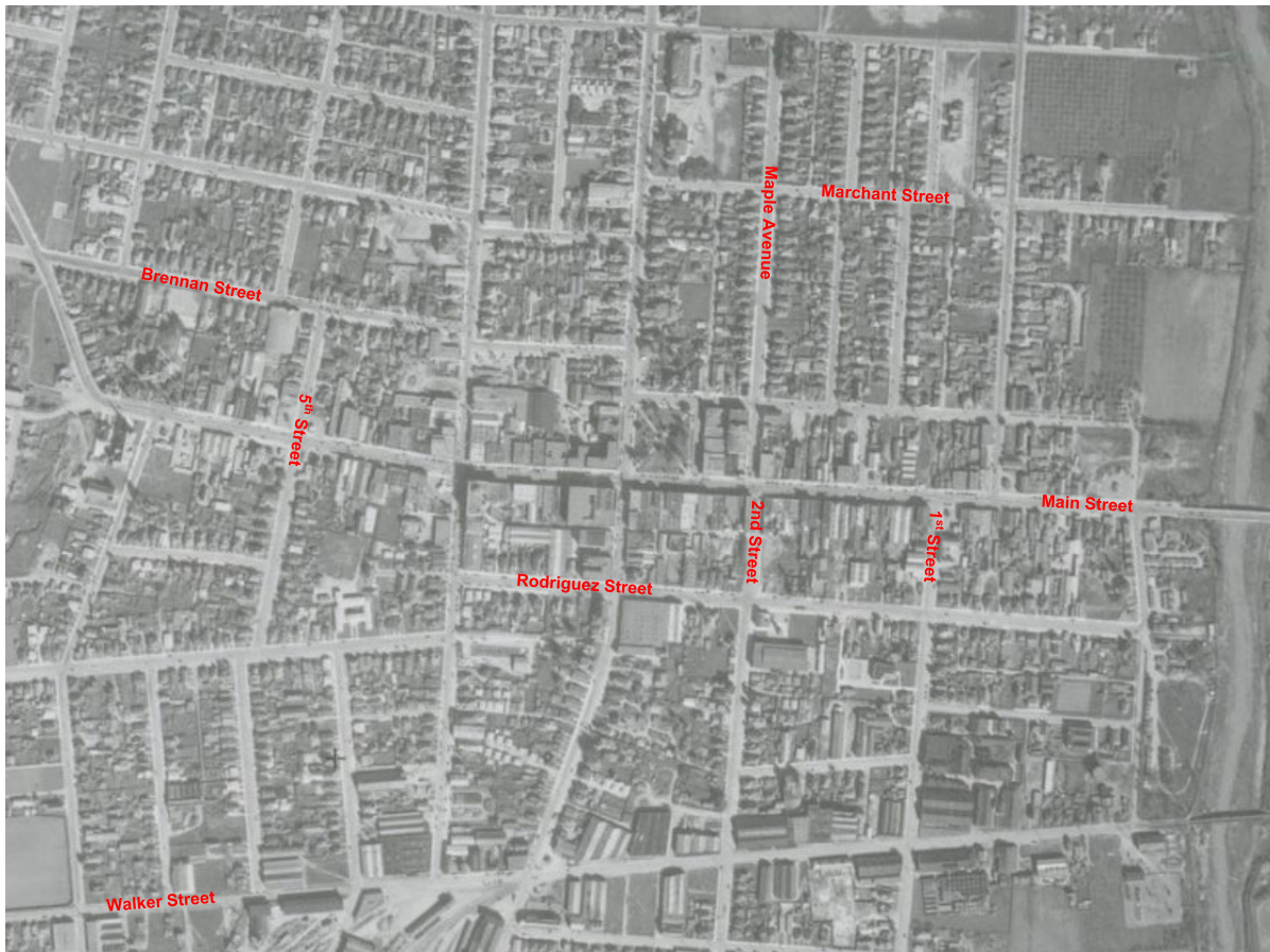
Figure 4.4-2 1935 Aerial Photograph of Downtown Watsonville
