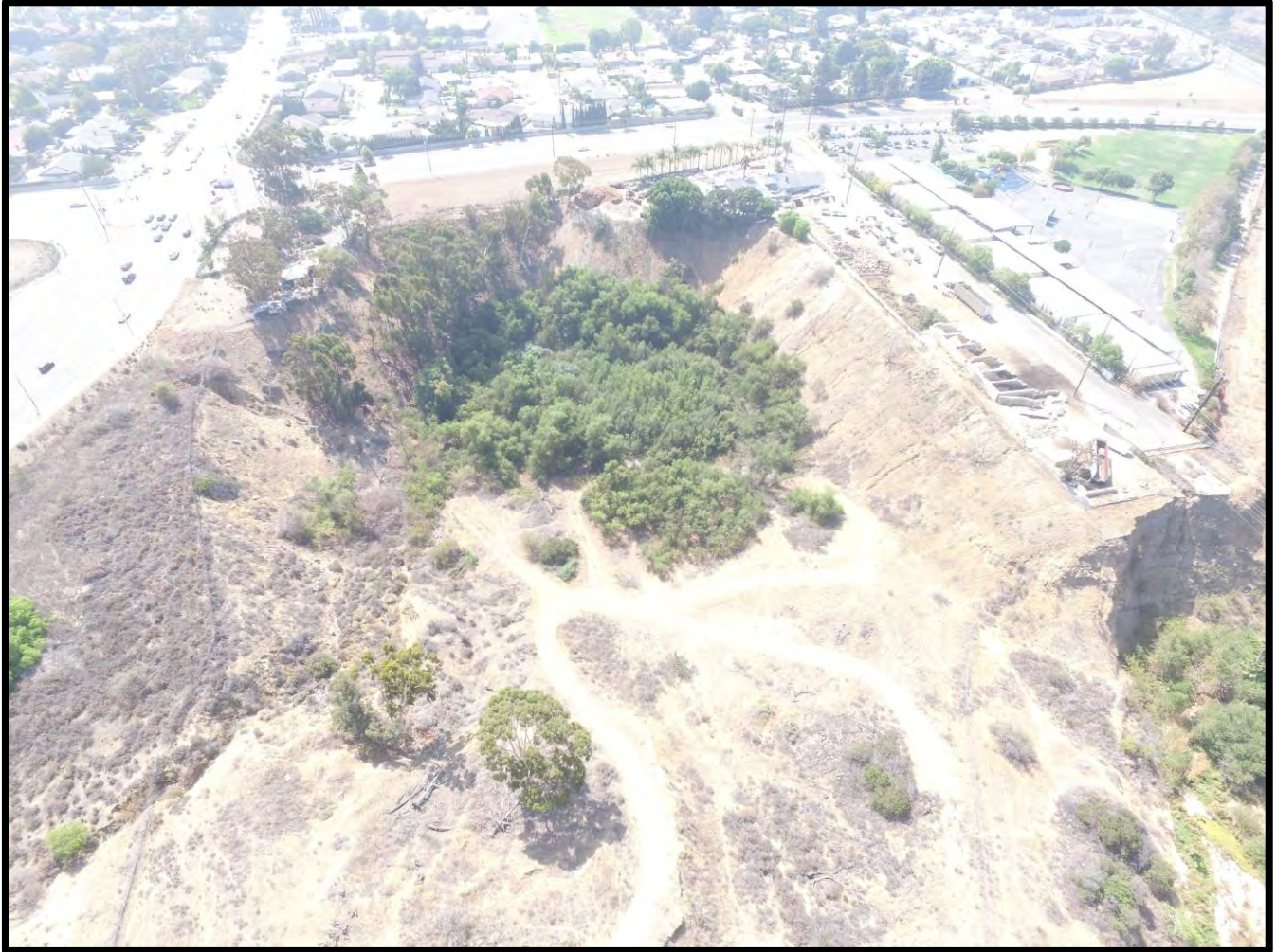
Aerial Photograph 3: Project Site/Access Roads - Looking South
