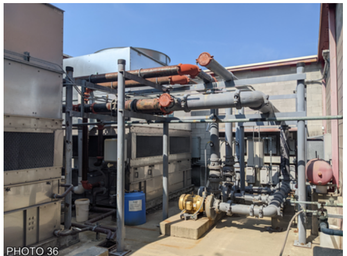
COOLING TOWER & PIPING
