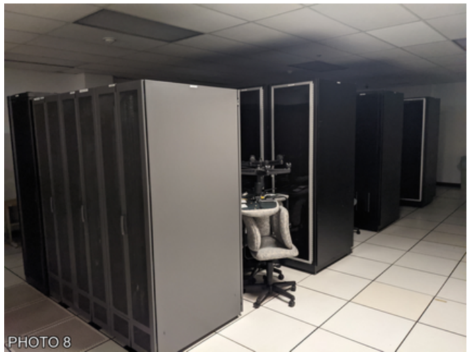
SERVER RACKS ON VENTED FLOOR
