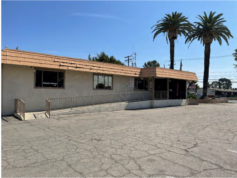
Photo 1: View of the office building on the northeast portion of the site, from the southwest.
