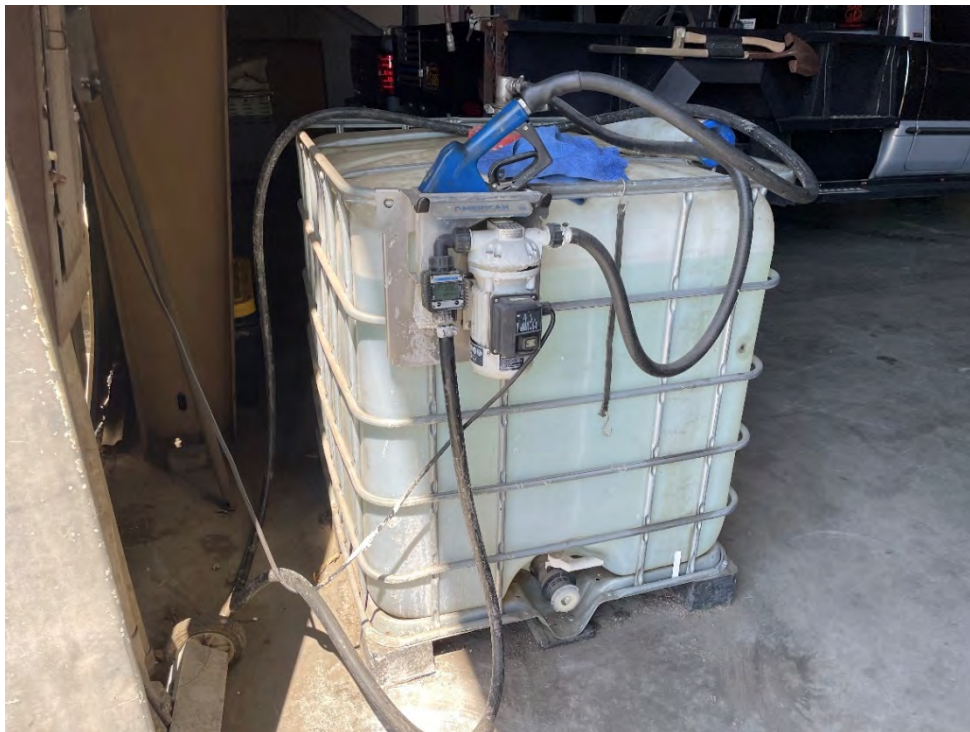
Photo 16: View of unlabeled tote with attached fuel pumping mechanism located in the southern portion of the warehouse.
