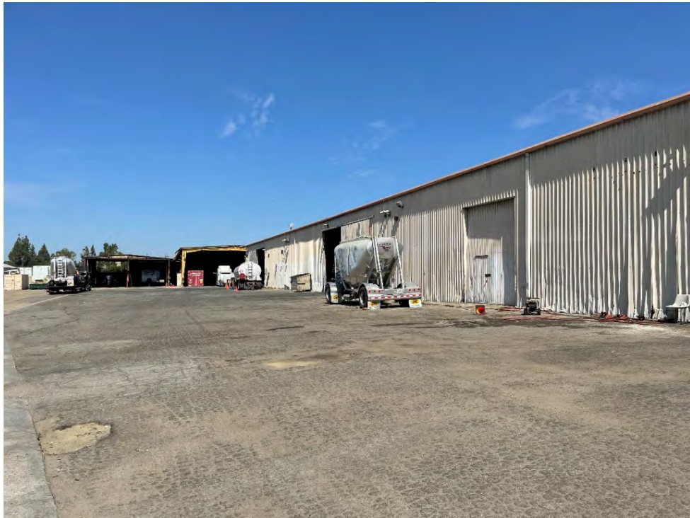
Photo 2: View of the warehouse located on the northern portion of the site (from the southeast) and two canopies in the northwest portion of the site (from the east).
