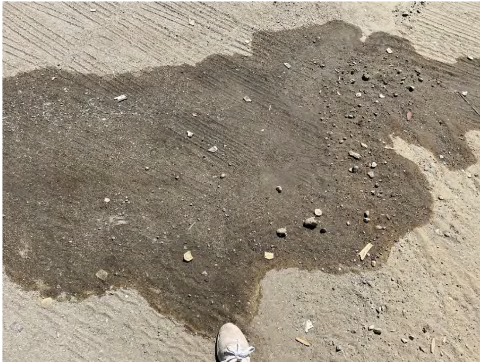
Photo 10: View of staining on unpaved surface located on the western portion of the site.
