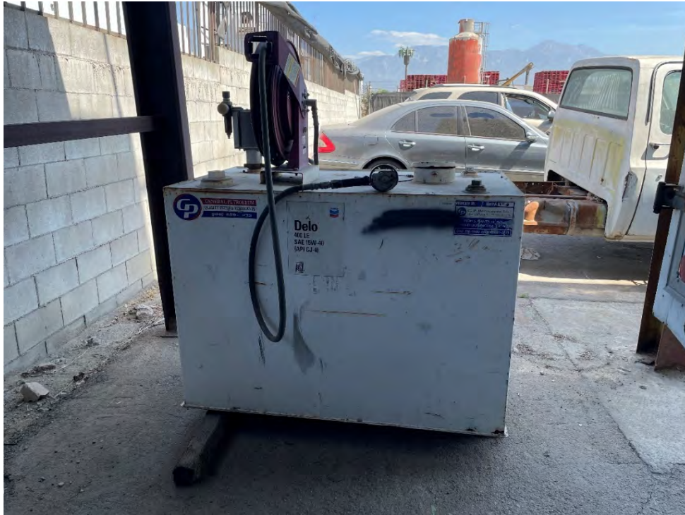
Photo 15: View of the engine oil AST located under the northern canopy on the northwest portion of the site.
