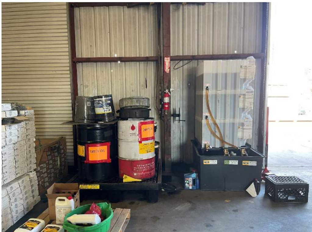
Photo 13: Hazardous waste storage area with used oil drums on secondary containment and new oil ASTs on secondary containment.
