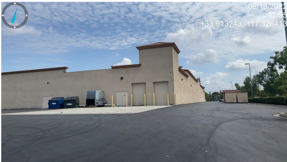
Photo 7: View Northeast of southern side of project site existing structure, also showing active recycling center structure.
