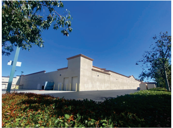
Photo 6: View from southwestern corner looking northeast.
