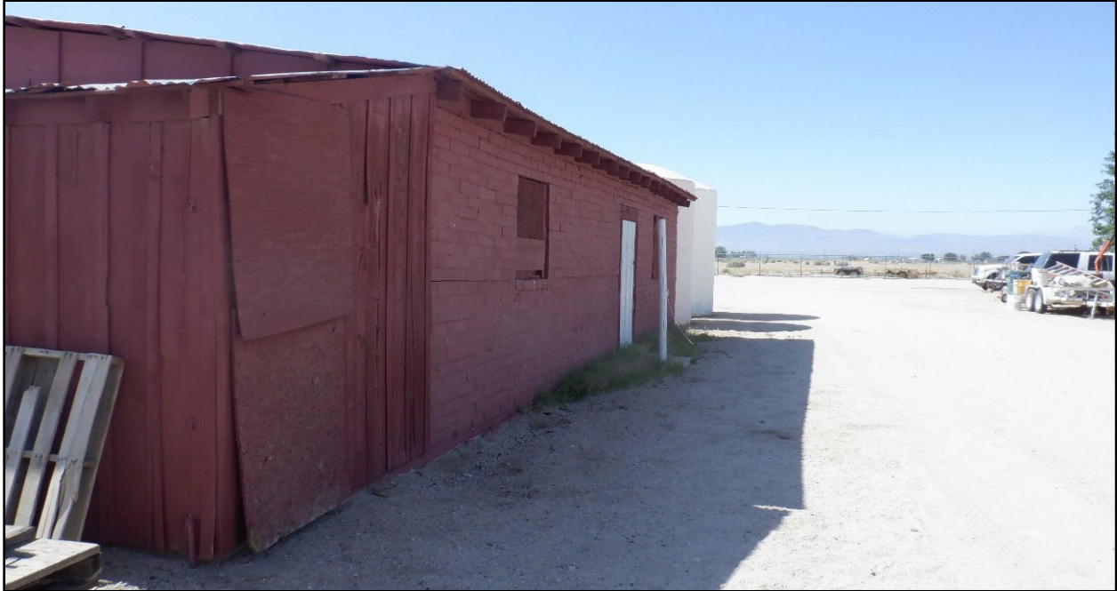
Photo 10: Building 5 (storage building), June 17, 2022 (view southeast).
