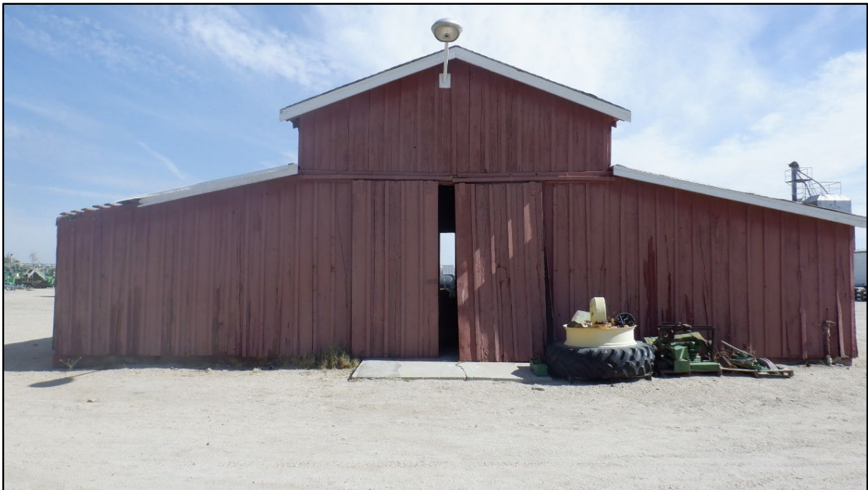
Photo 9: Building 4 (barn), June 17, 2022 (view north).
