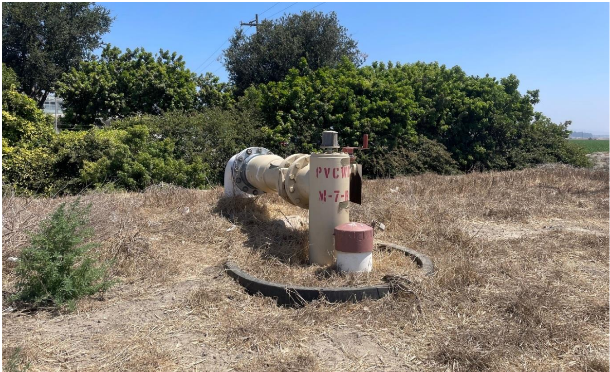
Figure 8 Underground Utility Within Project Site, Facing North
