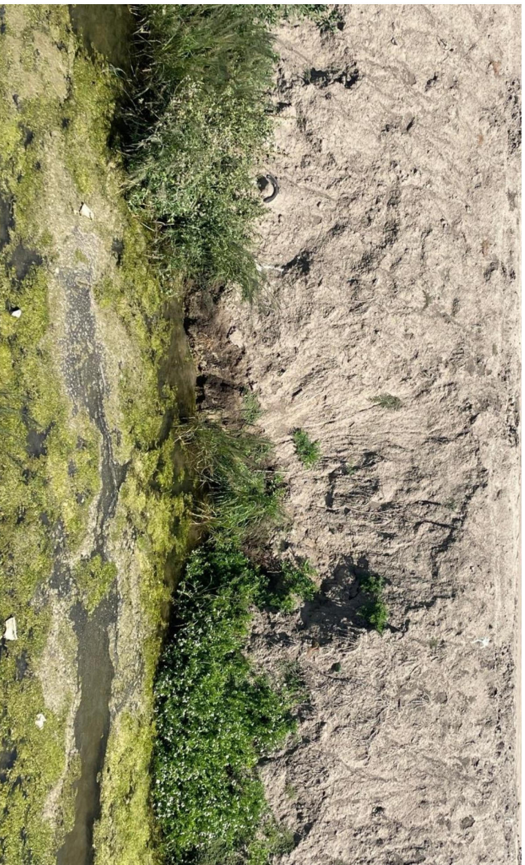
Figure 14 V-ditch Profile, Facing North
