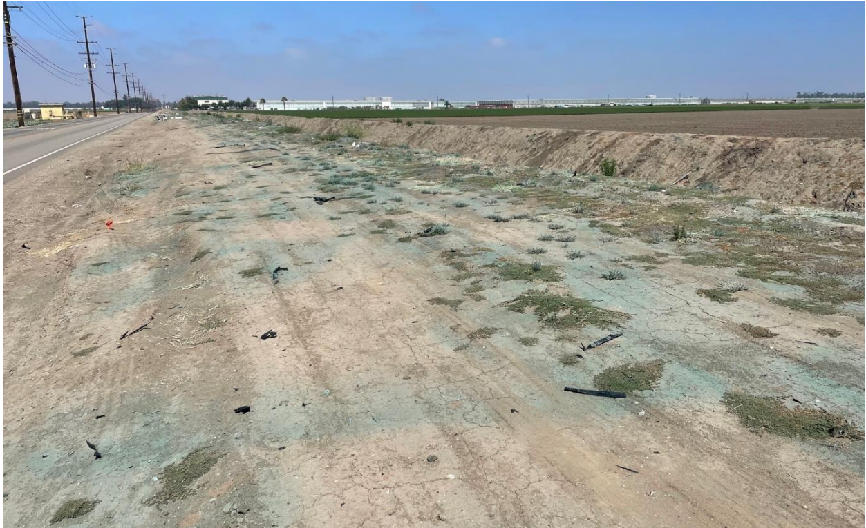
Figure 6 Soil Discoloration, Facing West
