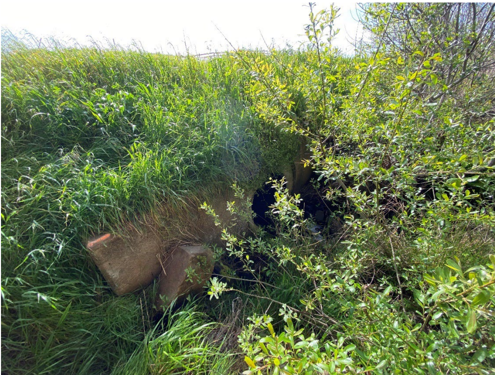
Photo 2. Culvert Inlet and Headwall
