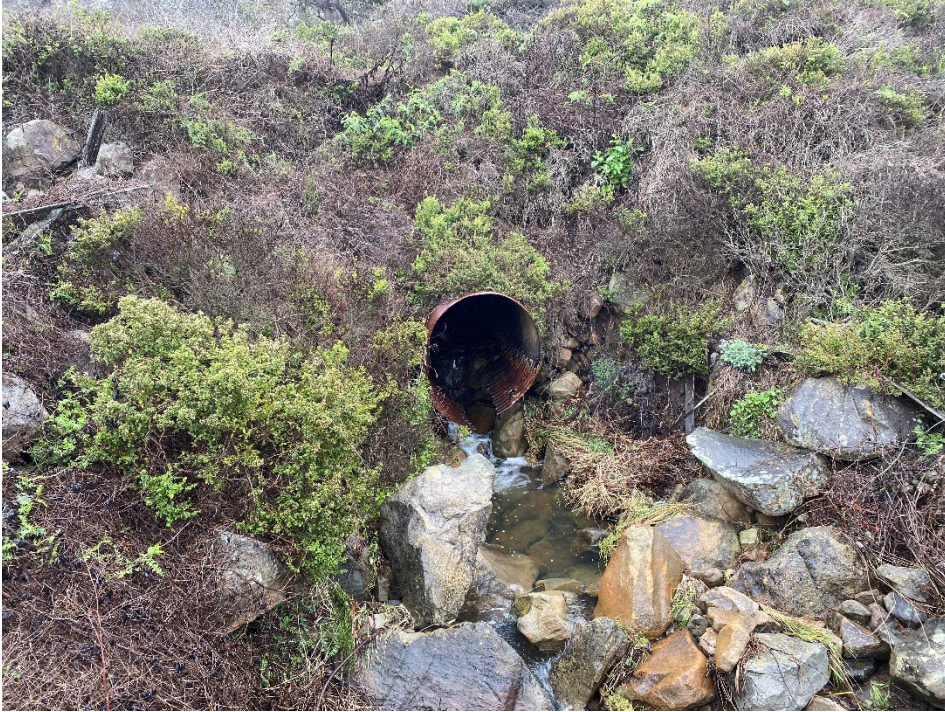
Photo 1. Existing Culvert Condition at the Downstream End
