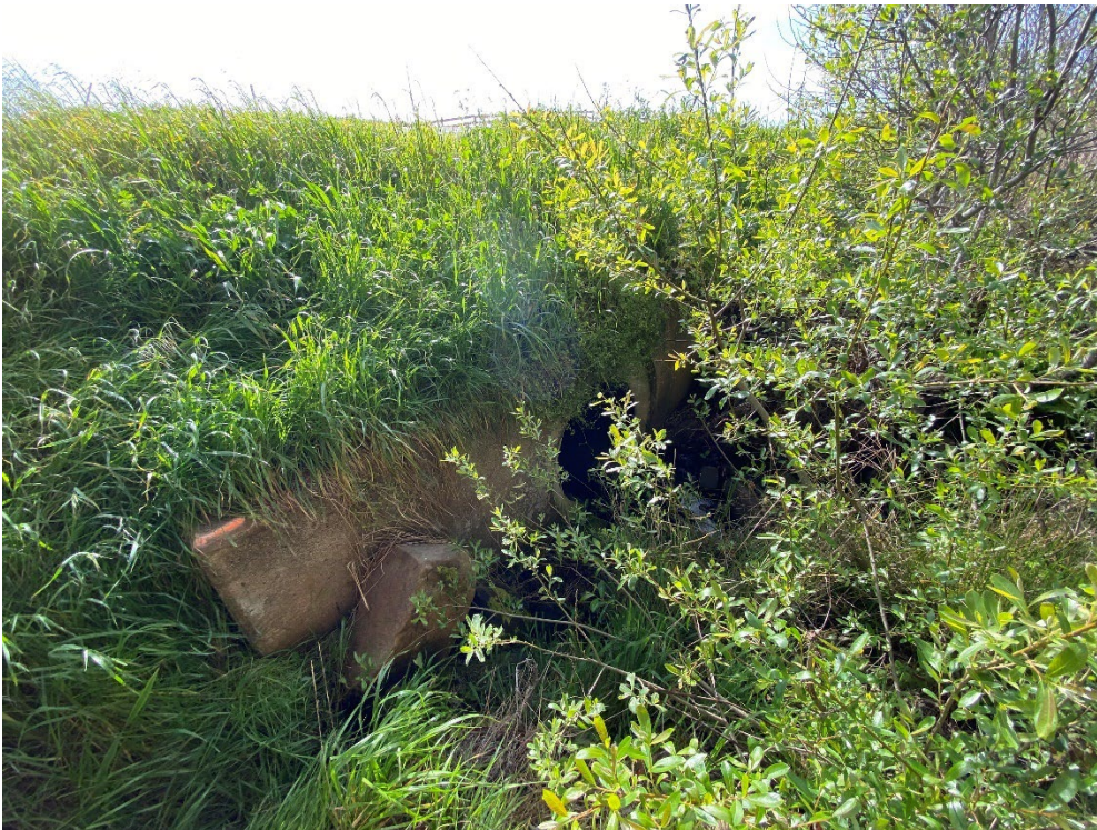
Photo 2. Culvert Inlet and Headwall
