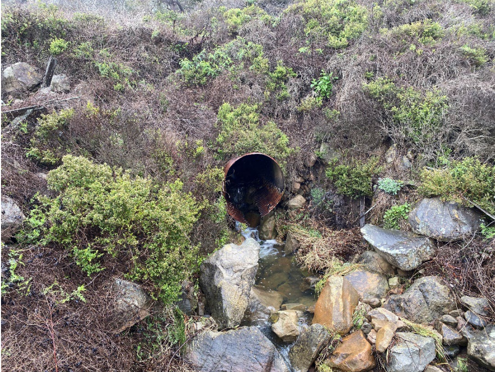
Photo 1. Existing Culvert Condition at the Downstream End
