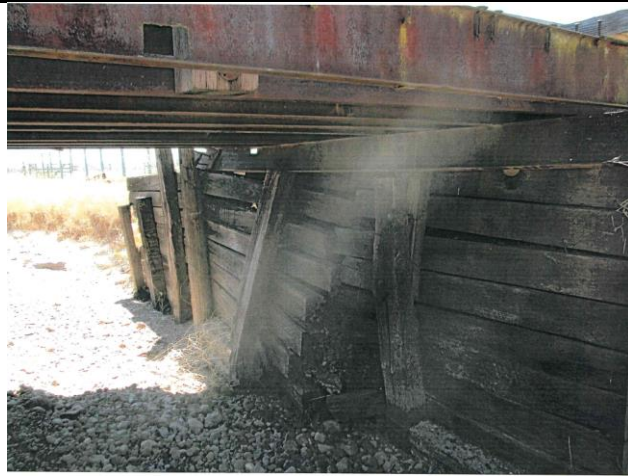
Figure 1 Substructure of bridge
