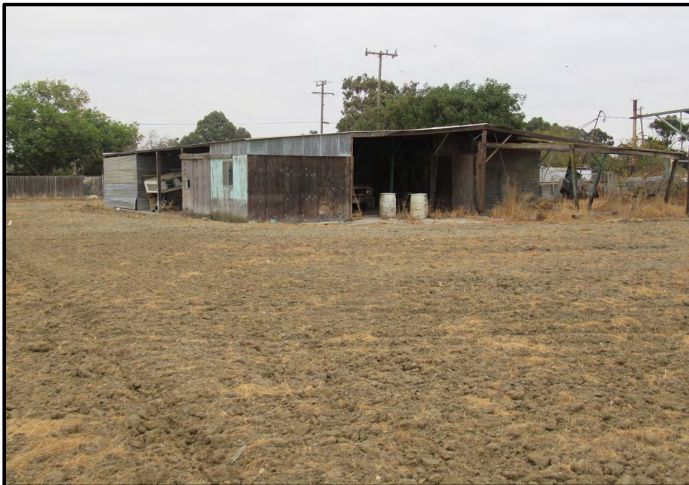
Close-up of the structure in the southeast part of the site, looking southeast; 05/13/22.
