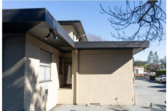
Figure 7: Easternmost portion of the south façade of 680 University Avenue. Looking north.
