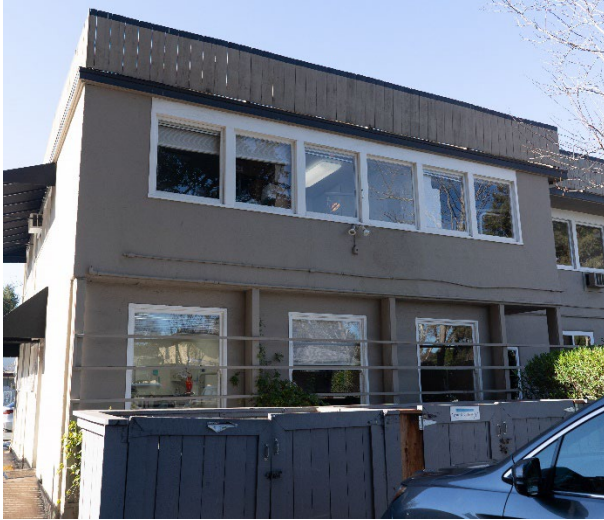
Figure 6: East section of rear façade. Looking southwest.
