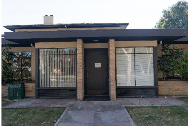
Figure 3: Primary entrance to subject building at west façade. Looking east.
