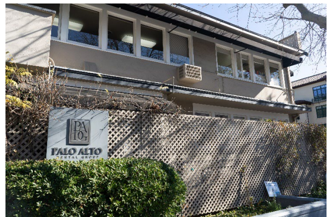
Figure 3: East portion of the first floor of the primary façade. Looking northeast.
