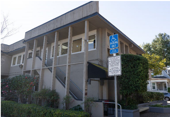
Figure 9: West section of rear façade. Looking southeast.
