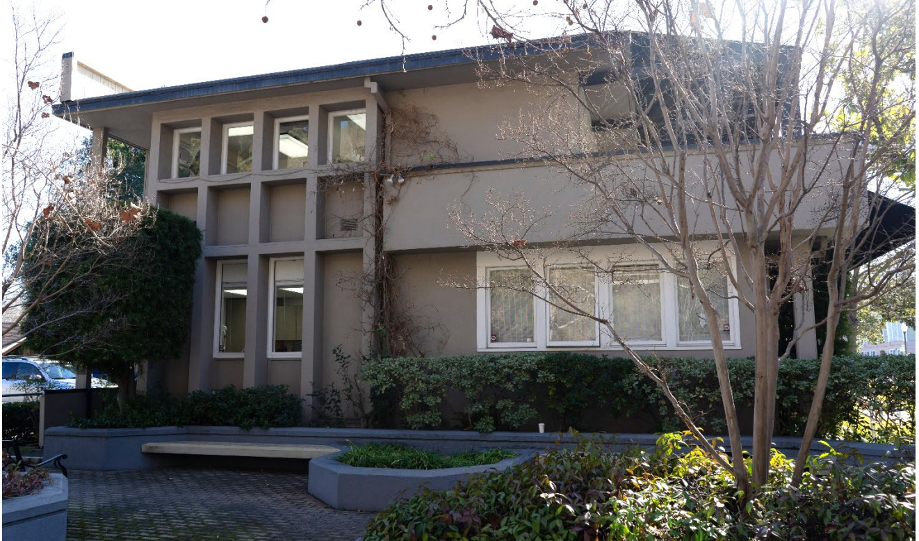
Figure 4: West façade of the subject building, looking slight northeast.
