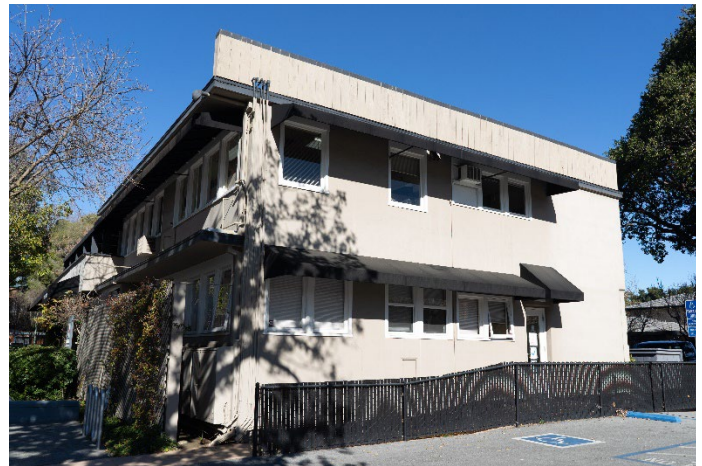
Figure 10: East façade of building. Looking northwest.
