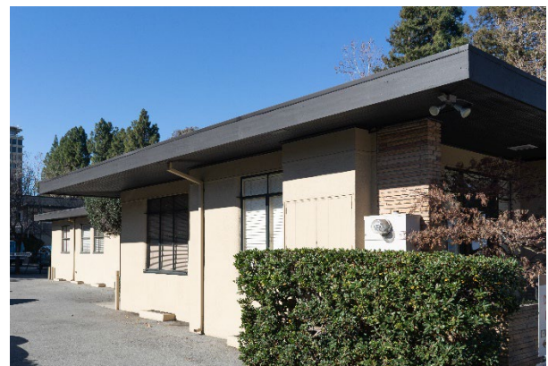
Figure 11: North portion of rear (east) façade of 680 University Avenue, looking southwest.
