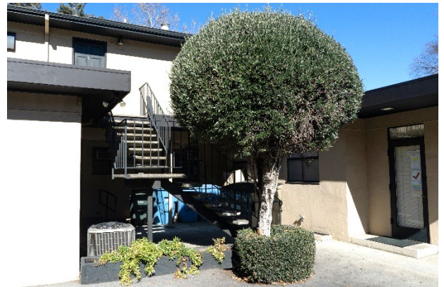
Figure 9: Central portion of rear (east) façade of 680 University Avenue, looking northwest.
