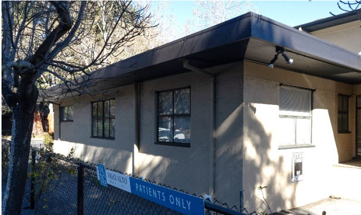
Figure 6: Westernmost portion of the south façade of 680 University Avenue. Looking northwest.
