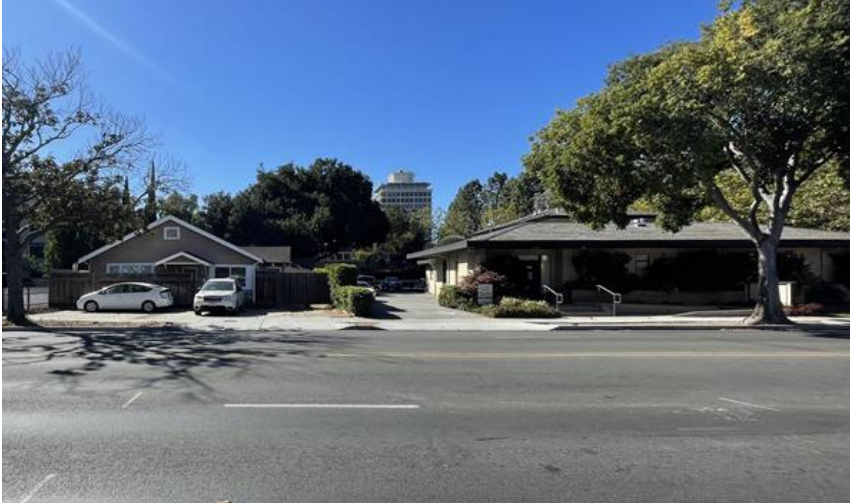
Photograph 3. View of the existing structure on the project site at 500 Middlefield Road (on the right side of the frame) from Middlefield Road looking southwest. The adjacent structure at 524 Middlefield Road is visible in the left side of the frame.
