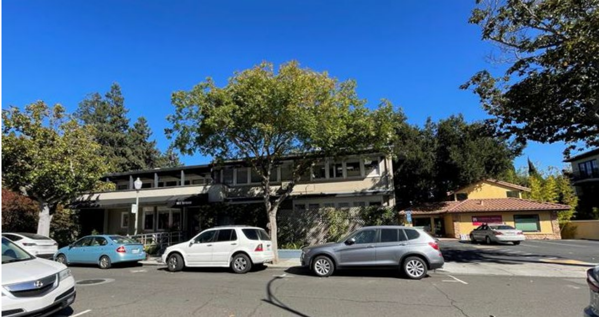
Photograph 1. View of existing structure at 511 Byron Street (on the left side of the frame), taken from Byron street, looking northeast. The adjacent structure at 517 Byron Street is visible in the right side of the frame.
