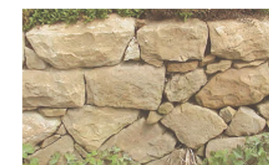
Santa Barbara Sandstone Dry-stack Wall
