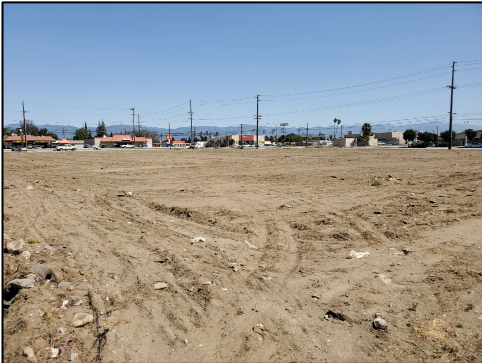
Plate 3.2-4: Overview of the project from the southwest corner, facing northeast.
