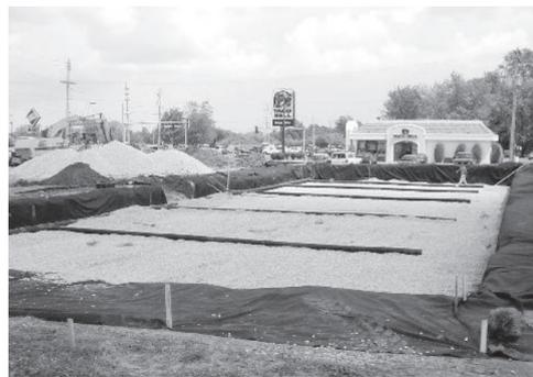
Place clean, crushed, angular stone foundation 9" (230 mm) min. Install underdrains if required. Compact to achieve a flat surface.
