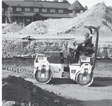
Install non-woven geotextile over stone. Geotextile must overlap 24" (600 mm) in, where edges meet. Compact at 24" (600 mm) of fill. Roller travel parallel with rows.
