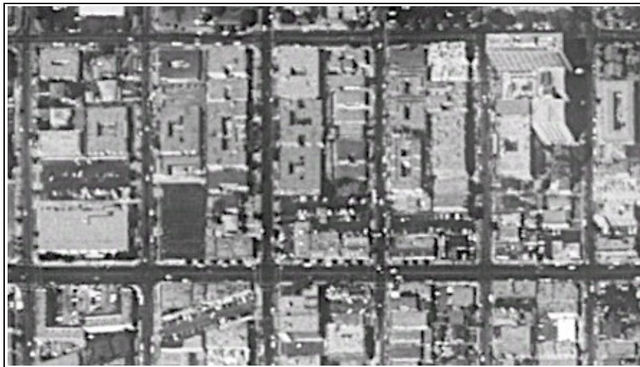
Figure 6: The Project area in 1989 image, showing the project property (center) fully developed (facing north, with 8 th Street below center) (UCSB Historic Aerial Image Database).
