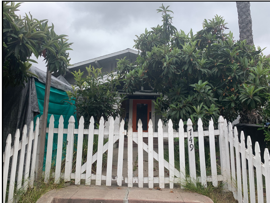
Figure 8: The Project Property, showing the front of the single family residence.
