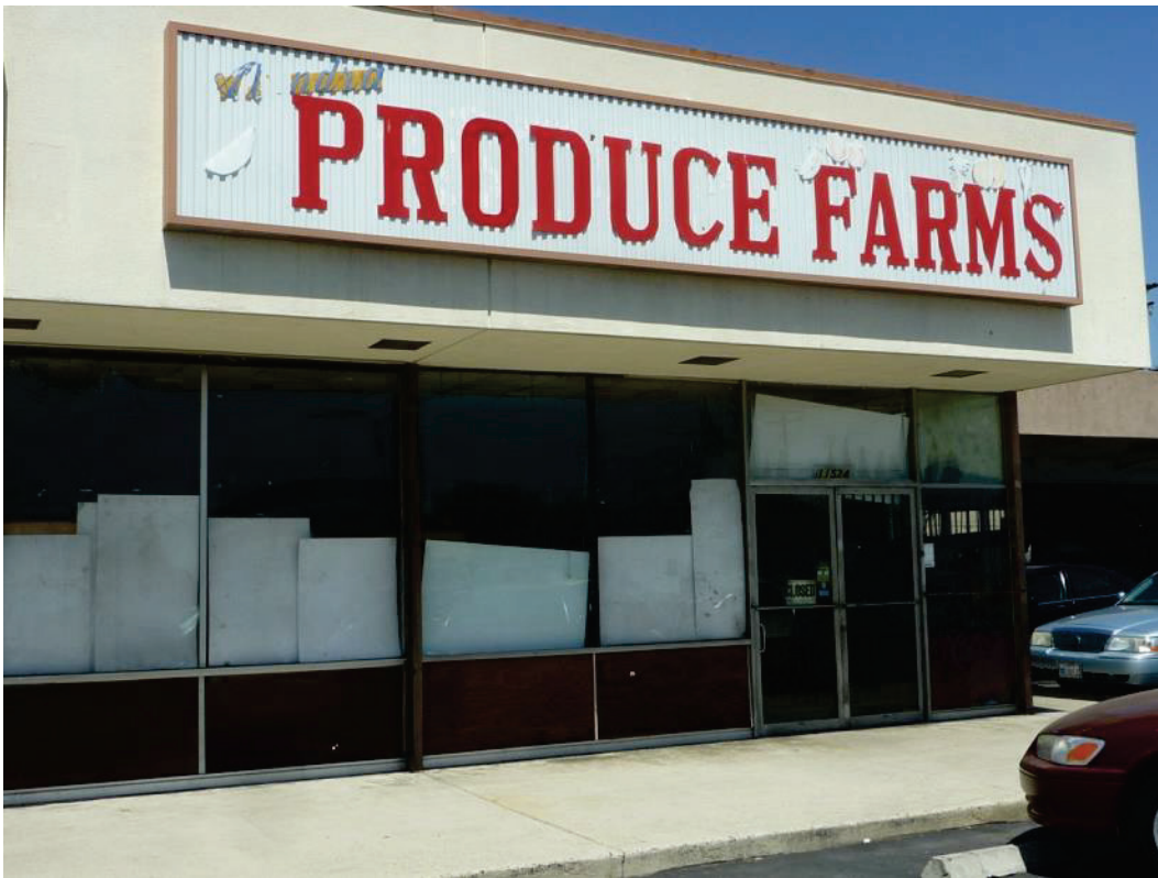
F-13. Exterior of former convenience store at 11524 Alondra (7/10/2014).
