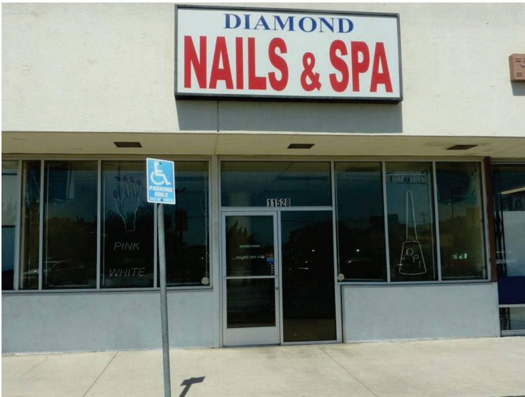
F-21. Exterior of former nail salon at 11528 Alondra (7/10/2014).
