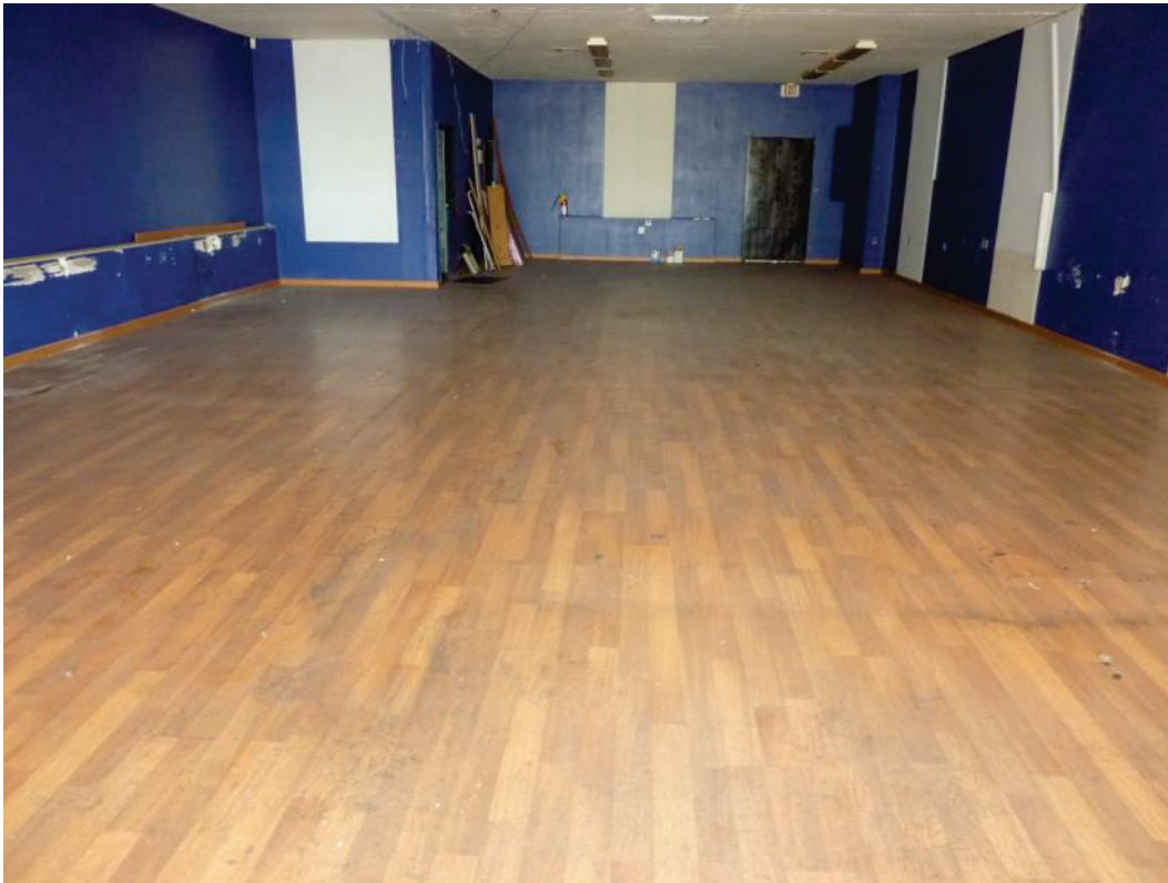
F-25. Interior of former PC repair shop at 11534 Alondra (7/10/2014).
