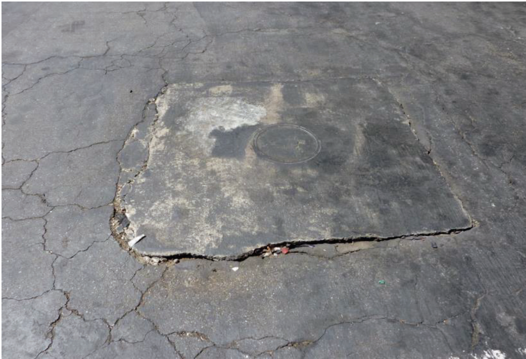
F-5. Possible former in-ground hydraulic vehicle lift outside Rusty's Automotive, 11522 Alondra (7/10/2014).
