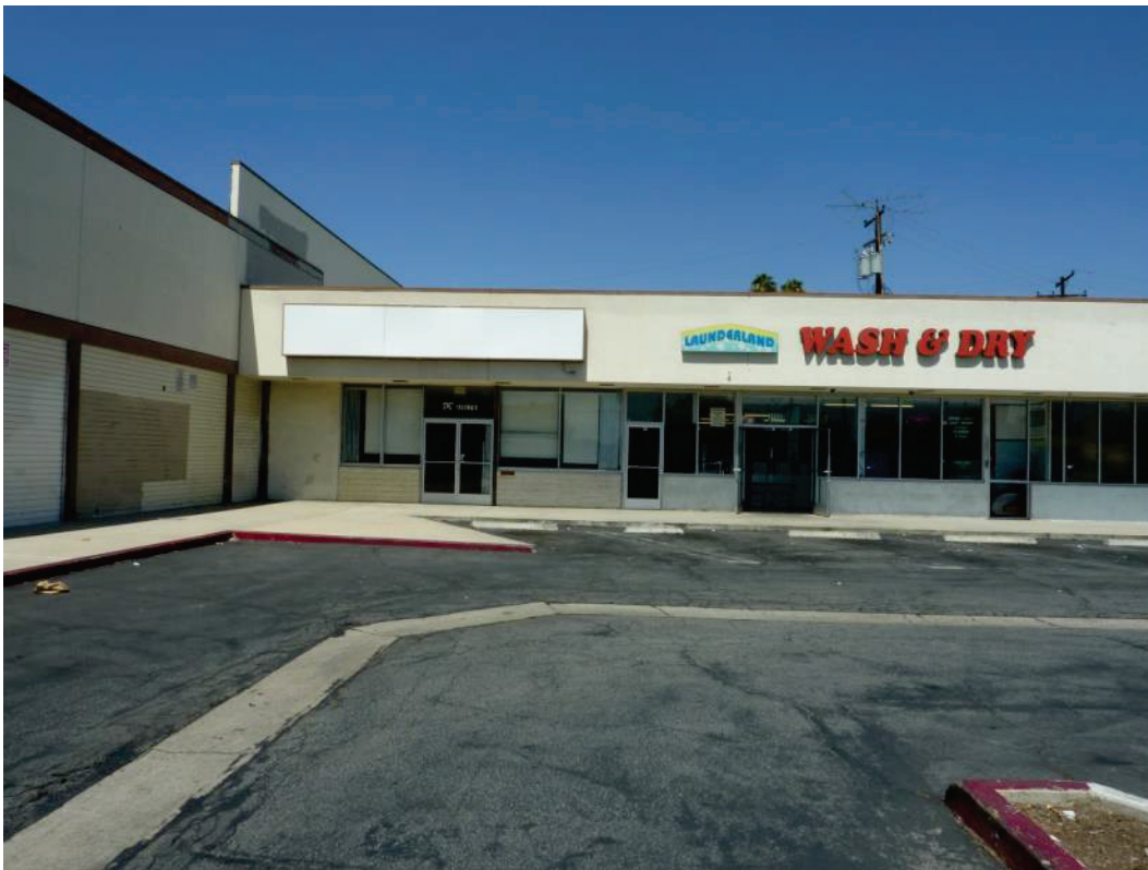
F-23. Exterior of Laundromat and former PC repair shop at 11530 & 11534 Alondra (7/10/2014).
