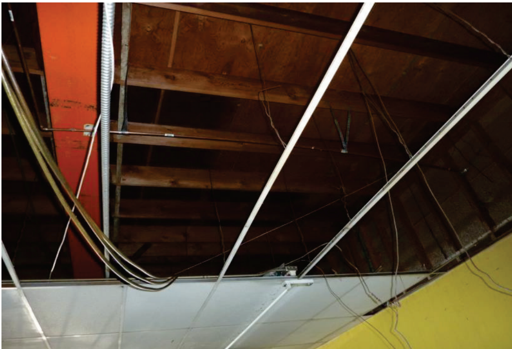
F-16. Exposed roof structure (uninsulated) inside former convenience store at 11524 Alondra (7/10/2014).
