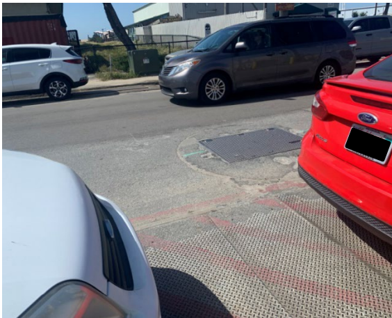
Photograph 3. Lift Station No. 3 Vault and Wet Well
