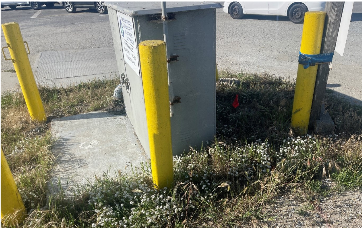
Photograph 4. Ruderal and developed land surrounding Lift Station No. 2, facing west. April 8, 2022.
