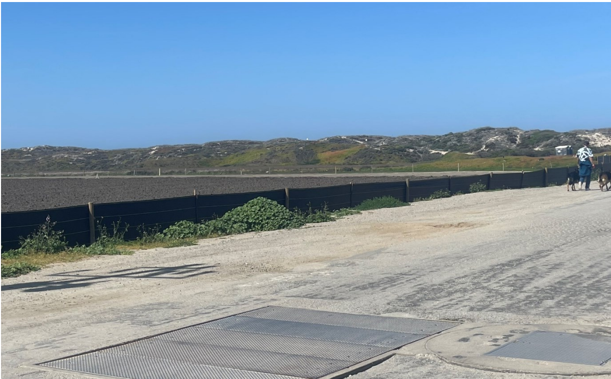
Photograph 6. Lift Station No 4 within the road (developed land cover) adjacent to cropland, facing southwest. April 8, 2022.
