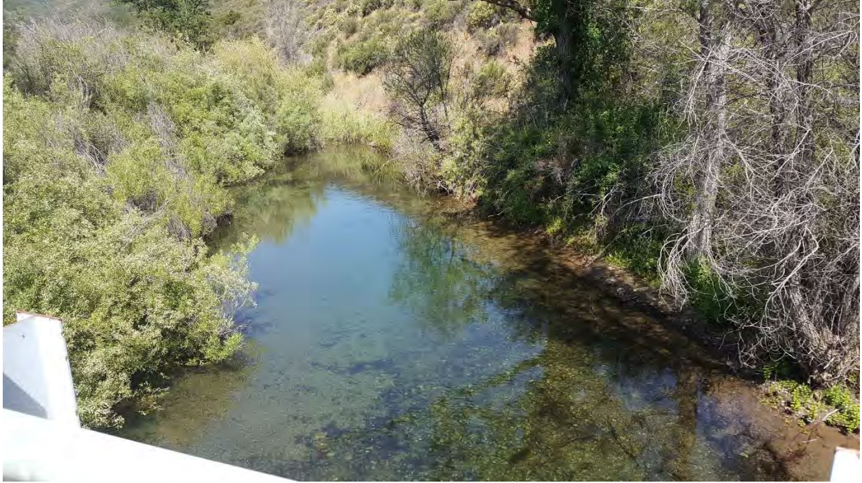
Standing on the Bartlett Springs Road bridge looking downstream at Bartlett Creek
