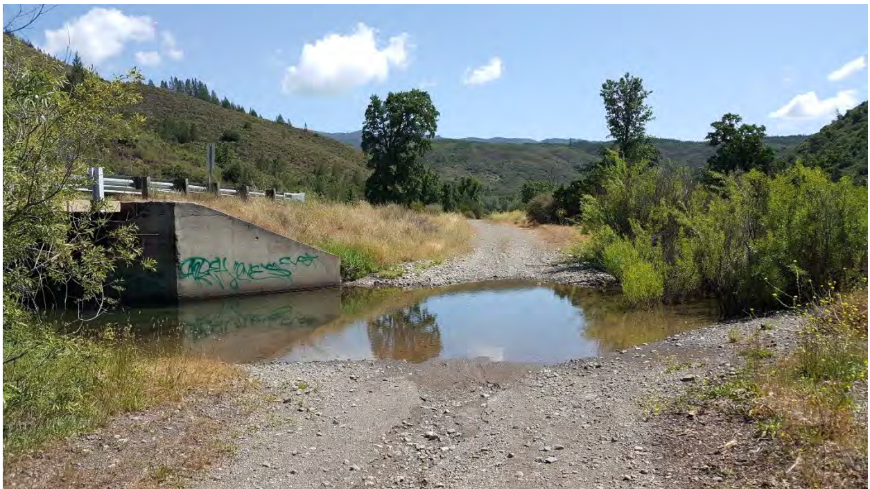
Standing on the low water crossing east of the existing bridge.
