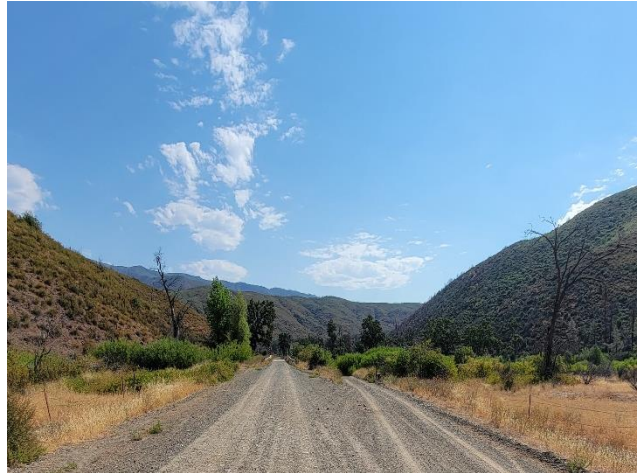
Photo 2: Standing in the northern portion of the project site looking southwest at the bridge.
