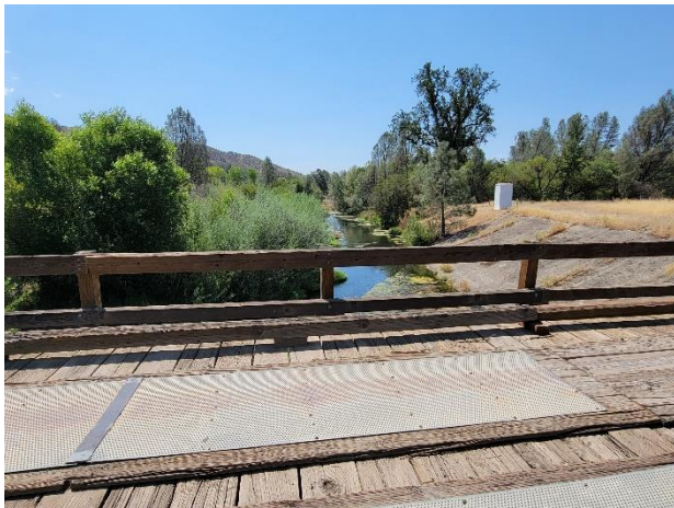
Photo 3: Standing on the center of the Chalk Mountain Bridge looking upstream.
