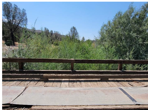
Photo 4: Standing on the center of Chalk Mountain Bridge looking downstream.
