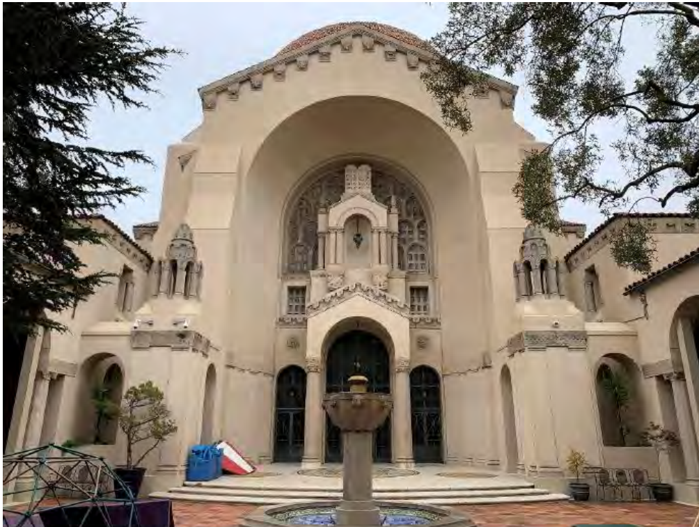
Courtyard, looking north at the south façade of the Sanctuary Wing. Brick paving in the foreground and the fountain at the center would be removed. Red arrow indicates location of new rectangular volume faced in bronze on the hip roof of the south wing flanking the Sanctuary Wing entry arch. Mark Cavagnero Architects photo, from HRE Part 1 by TreanorHL.
