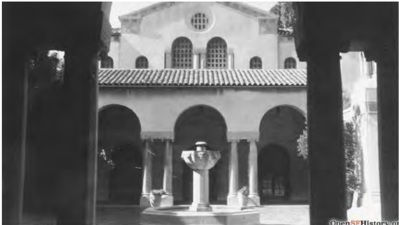
Courtyard, looking west with gable of main roof mass of the Temple House partially visible at top. The columns in the foreground and on the opposite side of the courtyard and the fountain would be removed, along with the cast stone screens over the two large level 4 windows of the Temple House, which would be replaced by a door and a window to provide access to the new roof deck and children’s play area. OpenSF photo, from HRE Part 1 by TreanorHL.
