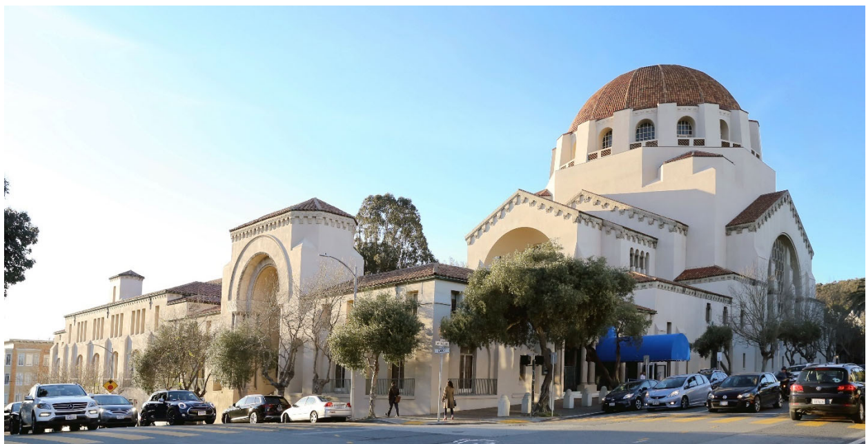
Figure 2. The south and east elevations of Temple Emanu-El, looking northwest from Arguello Boulevard (Mark Cavagnero Associates Architects).
