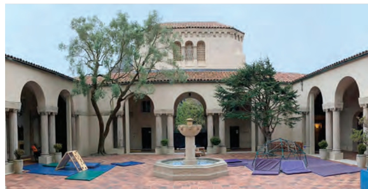
COURTYARD LOOKING SOUTH
