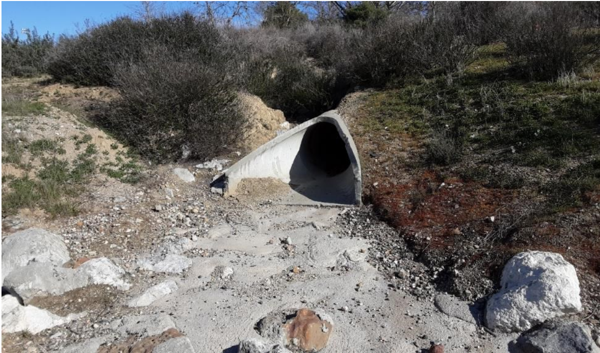
Photograph 10. Photo Point 10. View of Culvert Outlet 1 in the southern portion of the Study Area, facing northwest. Note concrete rip rap to the south (below) the outlet (February 23, 2022).
