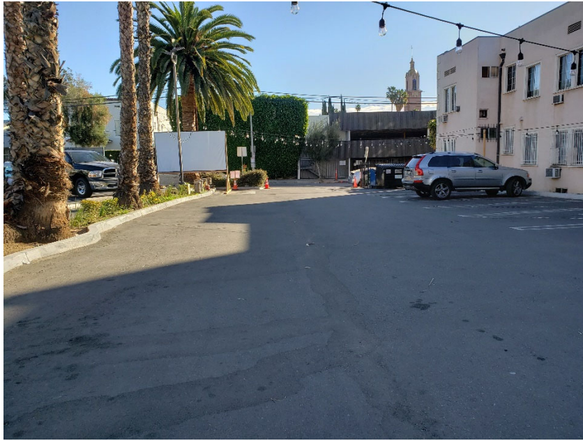
1. Asphalt-paved parking lots
