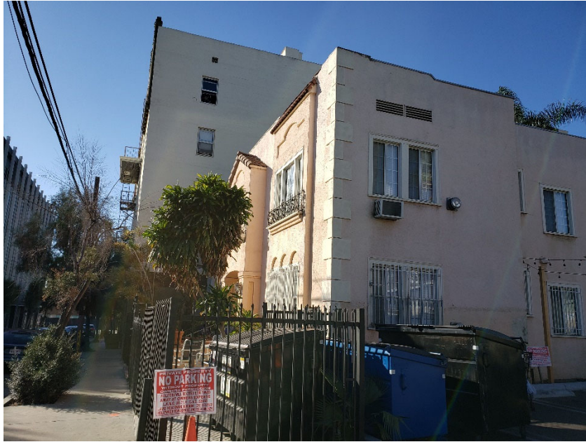
13. Adjoining property to the east
