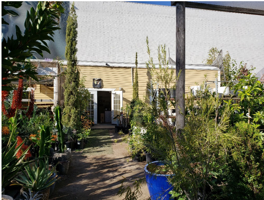
10. Temporary structure at 6751 Sunset Boulevard
