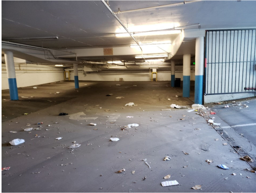
7. Below-grade parking level at 6767 Sunset Boulevard
