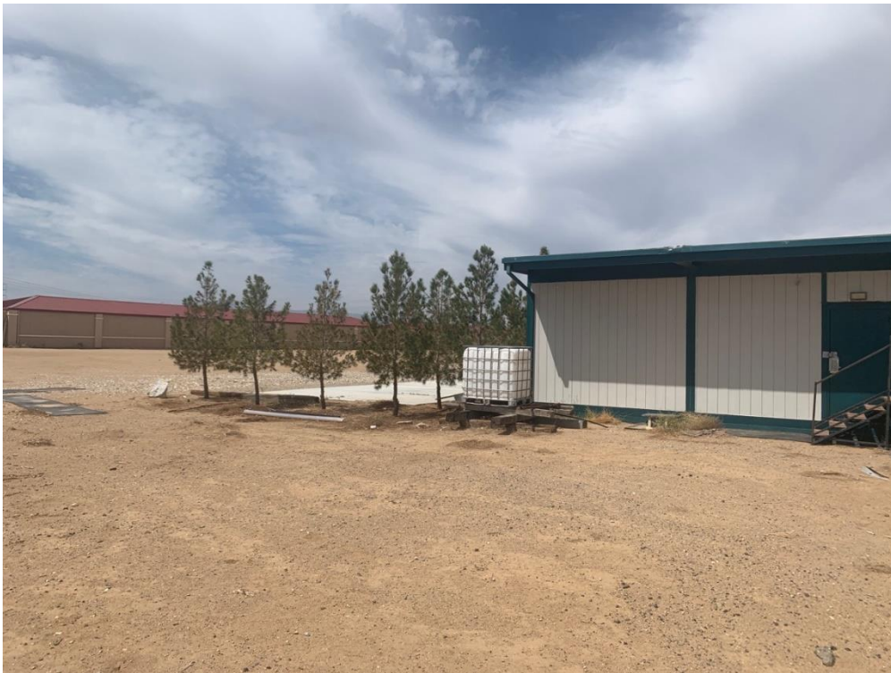
Photo 4. Photo showing the ornamental vegetation and building located in the northeast section of the site. Photo is facing southwest.
