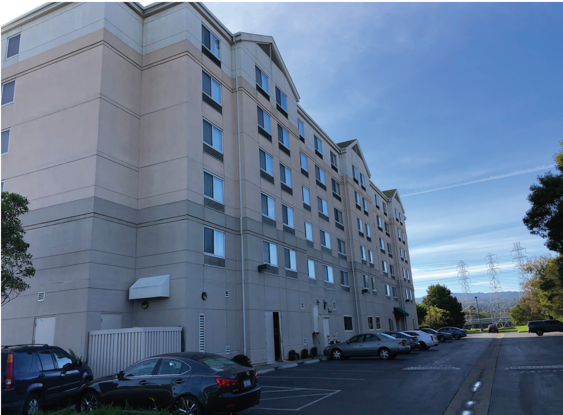
Photo 4: View of adjacent hotel building east of project site.
