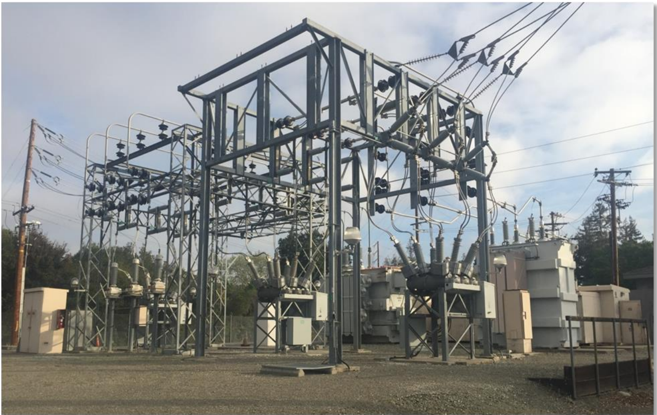
Existing Homestead Substation
