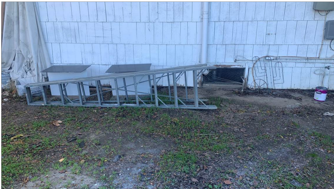
Photo 18: Opening to the underground of the house. Utility lines access.
