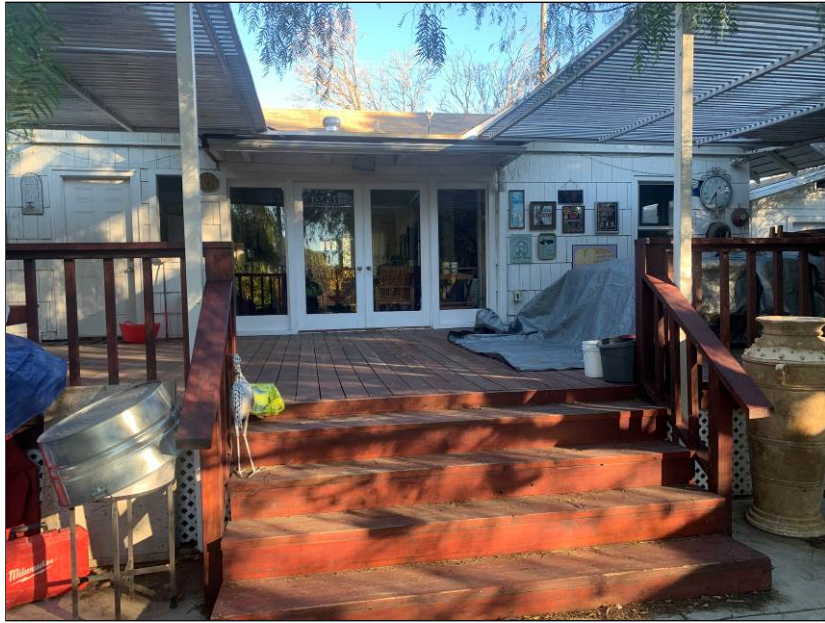
Photo 15: North facing backyard porch of the occupied residential structure.
