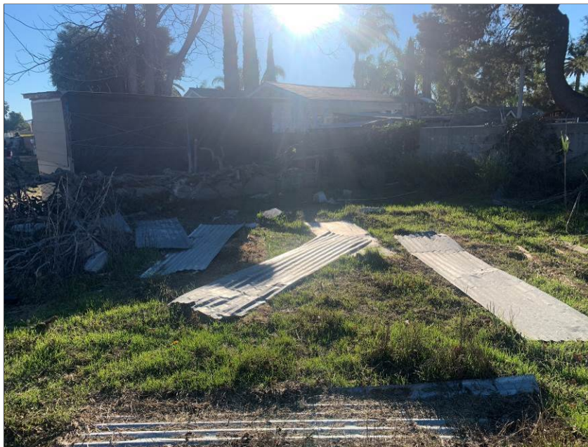
Photo 10: Southeast corner of the Site has some branches that seems to have damage the fence dividing the Site and the 15516-neighboring property.
