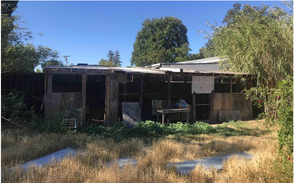
Photograph 6. Existing shed structure on the eastern parcel of the Project Site.
