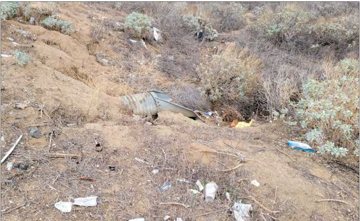
Photograph 8: View of eastern downstream outlet of Drainage 1 culvert, downstream and east of Moreno Beach Drive. Photo depicts existing 30" corrugated metal culvert which will be replaced with an appurtenant facility which includes an energy dissipater, headwall, rip-rap, 18-inch storm drain, and metal culvert.
