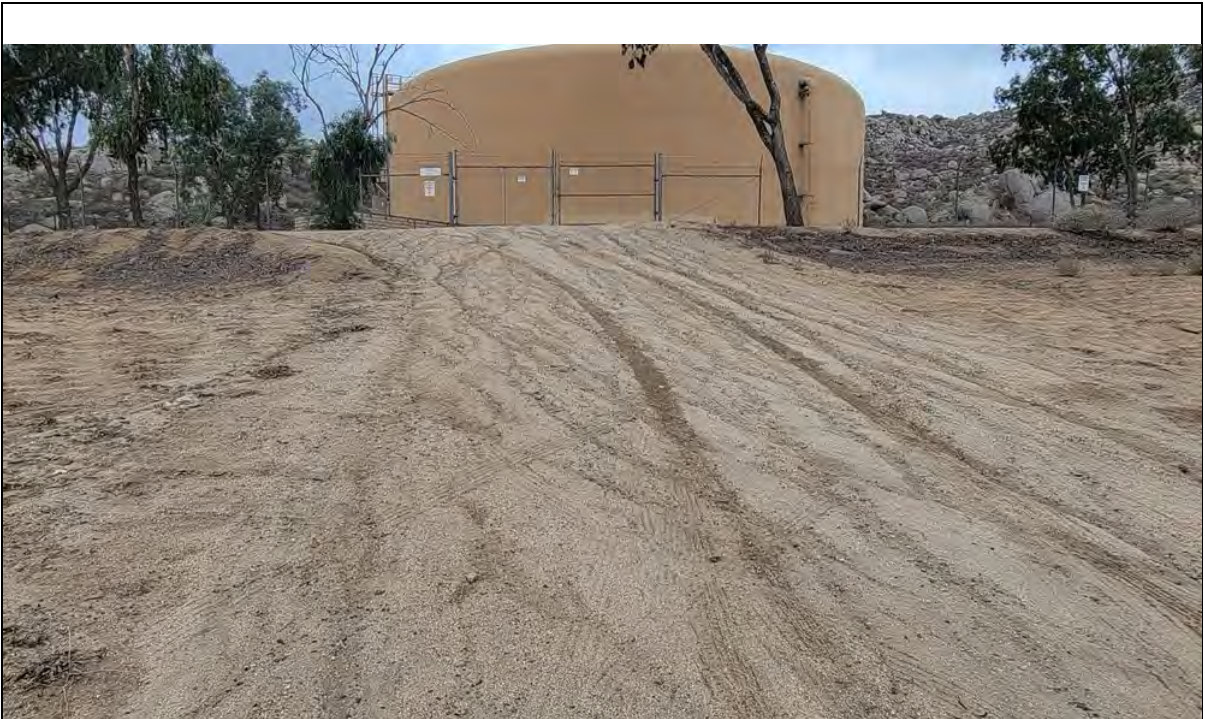
Photograph 1: View of east side of existing Pettit Water Storage Tank and entry gate, facing west. Photo depicts unpaved driveway and location of proposed transmission pipeline.
