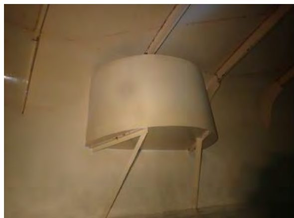
Figure 9: Overflow weir in good condition
