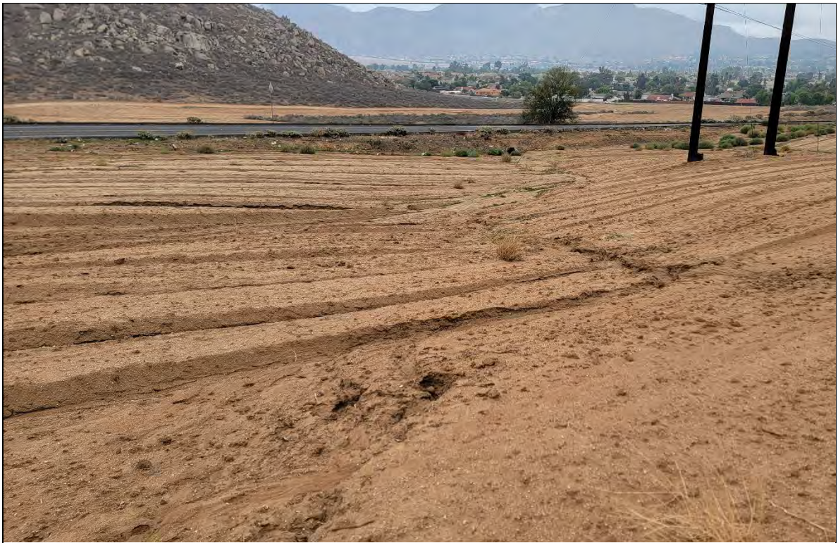
Photograph 13: View of erosional feature EF3 facing downstream and southeast from its northern terminus, towards its intersection with Moreno Beach Drive.
