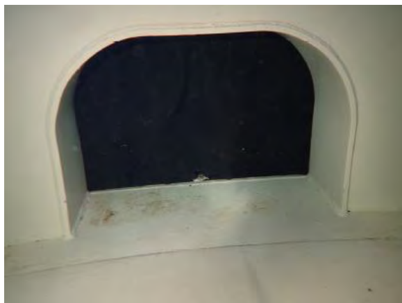
Figure 8: Doghouse-style drain through wall with no corrosion
