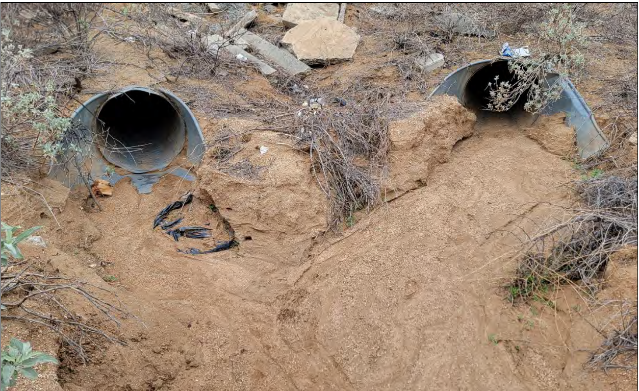
Photograph 12: View upstream towards two 30" culverts for Drainage 2 (left) and Drainage 3 (right), and their confluence just east of Moreno Beach Drive, facing west. Channel continues as a single drainage (Drainage 4) conveying flows to the east and southeast.
