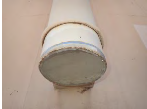
Figure 21: Overflow pipe in good condition
