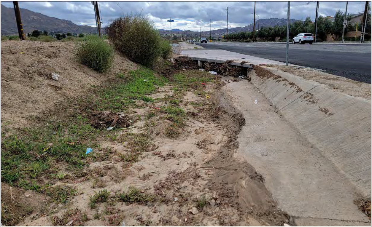
Photograph 15: View downstream and south of concrete lined channel portion of Drainage 4 where it enters a box culvert beneath Bay Avenue.
