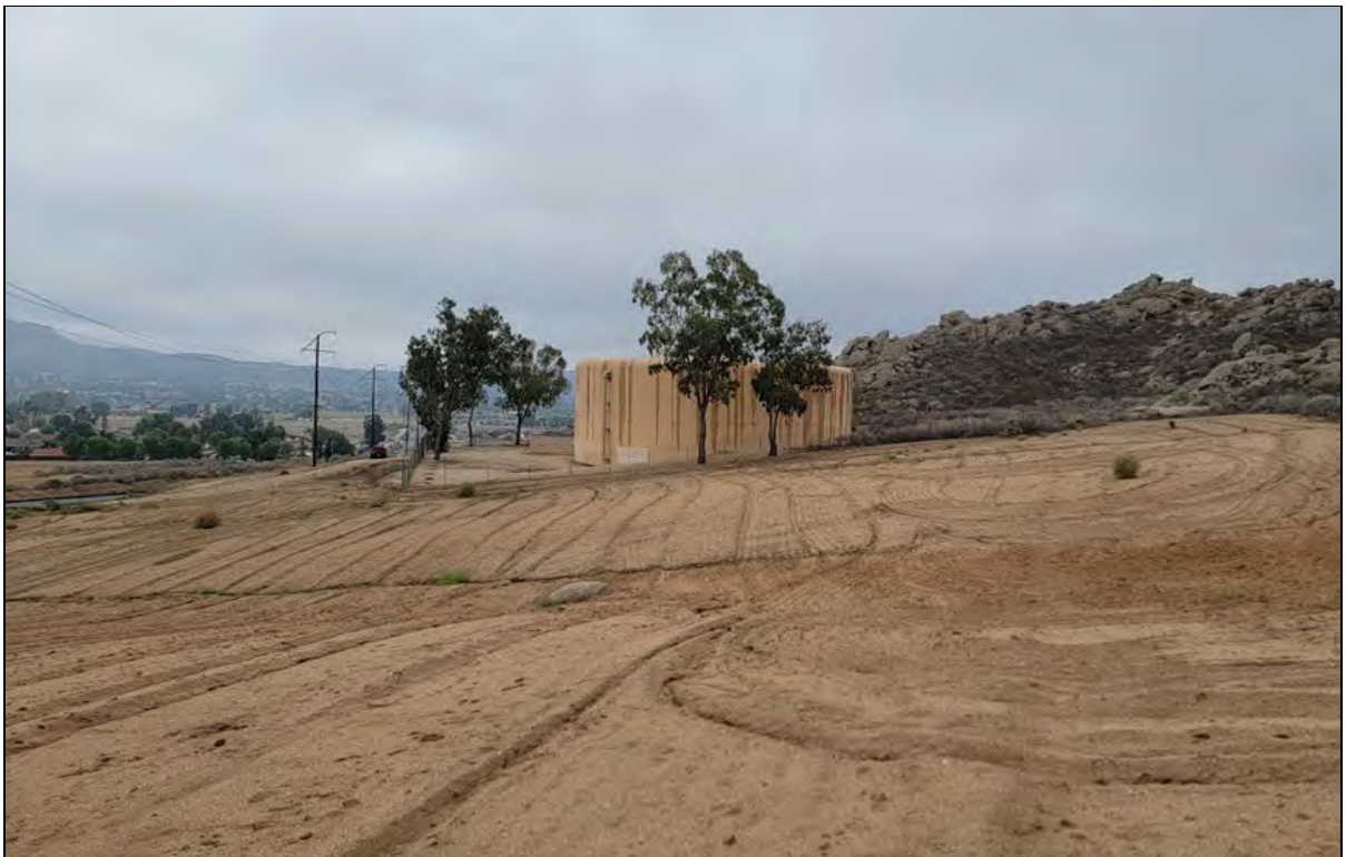
Photograph 6: View of Phase 1 water storage tank location, facing south from northern boundary of proposed grading limits. Photo depicts disturbed land north of the existing Pettit Water Storage Tank and brittle bush scrub west and south of the existing Pettit Water Storage Tank.
