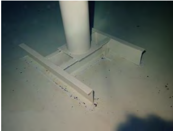
Figure 11: Column base in good condition
