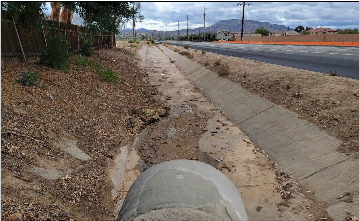
Photograph 14: View downstream of Drainage 4 from concrete culvert into 5-foot wide concrete lined channel portion, facing south along Moreno Beach Drive.
