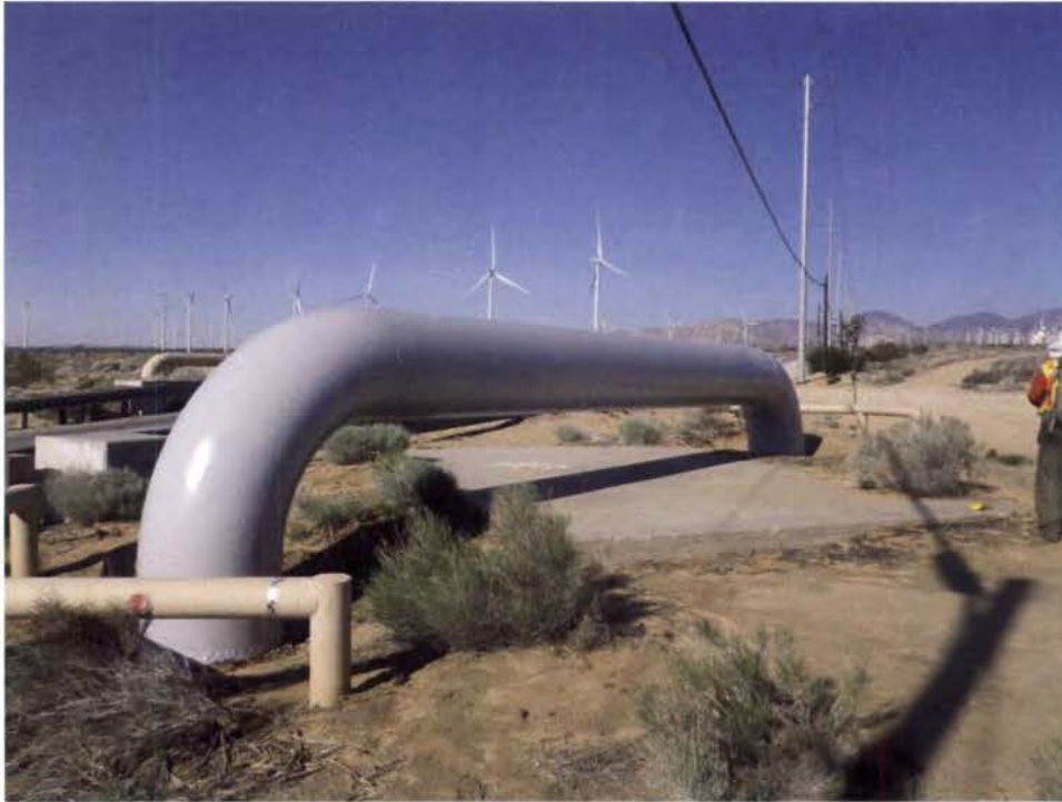
Folder: Rotation 1 Optio 35 File: IMG1935 PG&E pipeline crossing aqueduct, view to the west (View: west)
