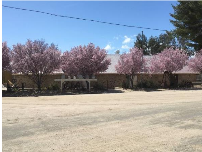
Photograph 4. Primary (north) elevation of Building H2 (the grocery store), looking south
