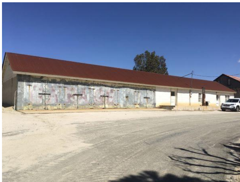
Photograph 5. Primary (south) elevation of Building H3 (the saloon), looking northeast
