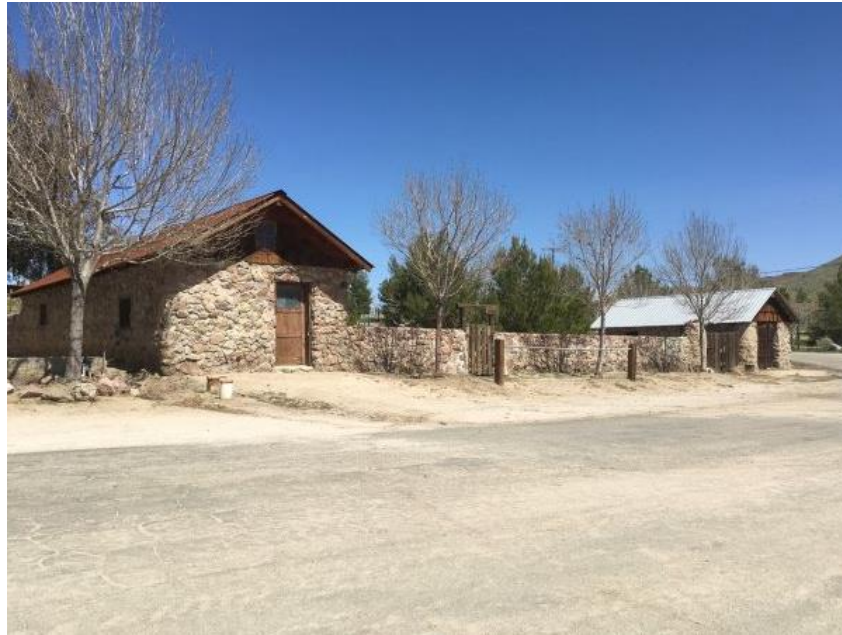
Photograph 6. Overview of Buildings H5 and H6 with stone and mortar enclosure, looking northeast
