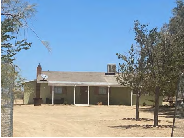
House 1 primary south elevation, facing north
