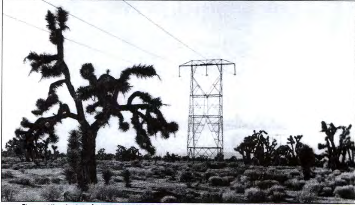
Figure 1: Historic view of a Suspension Vincent Tower. Image Source: Iron Men and Copper Wires (page 220).
