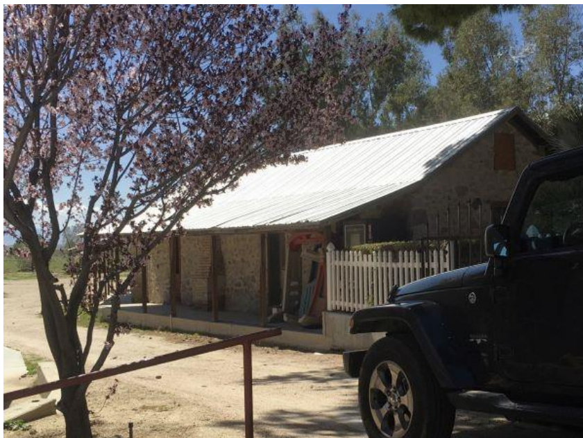
Photograph 10. Primary (east) and north elevations of Building H11, looking south
