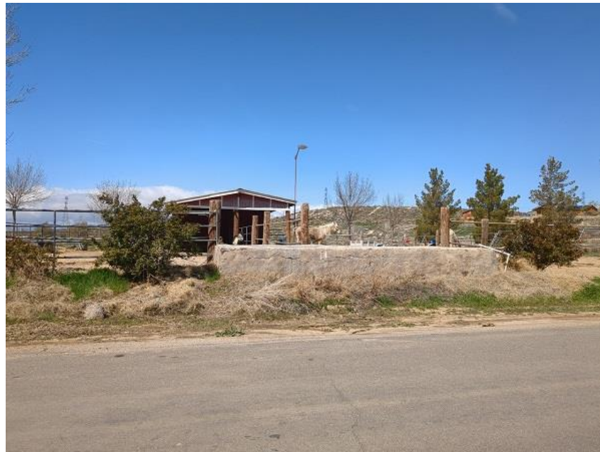
Photograph 2. Concrete and stone trough located south of 1937 CHL plaque, looking west
