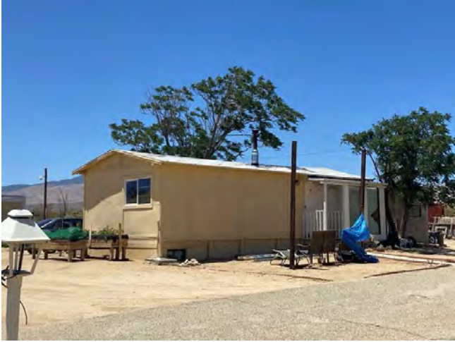
West manufactured home, south and west elevation, view facing northwest;
