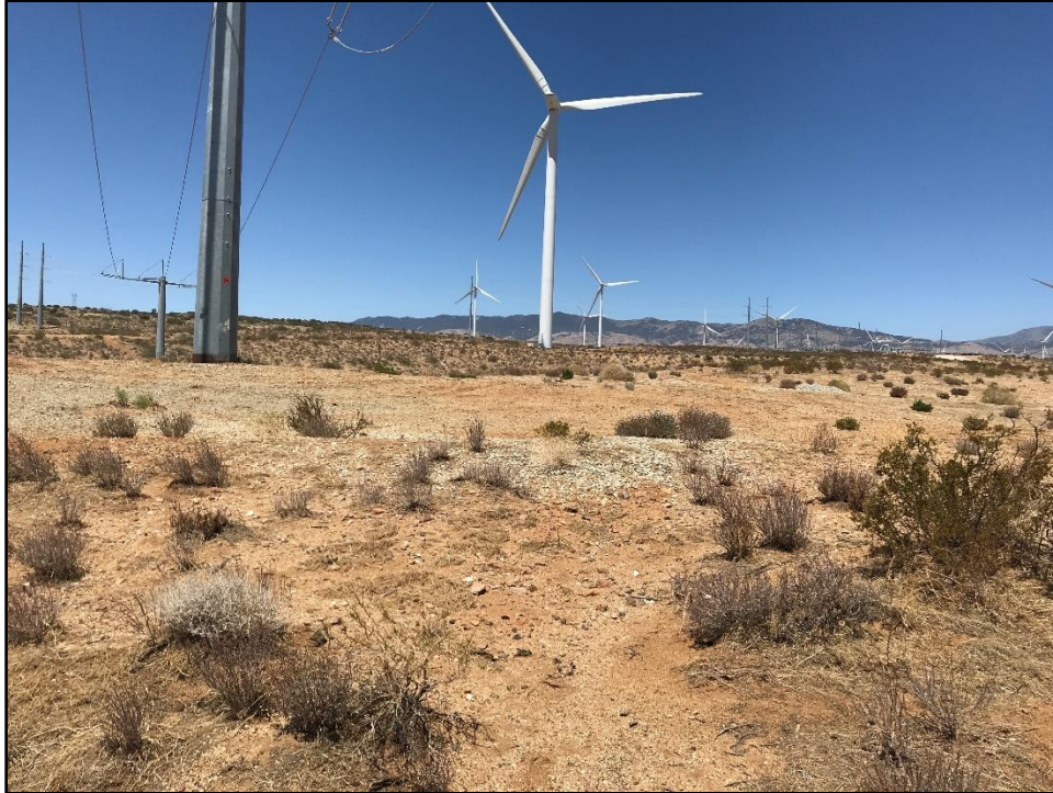
Figure 5. Photo taken from along gen-tie Whirlwind Option 1 (AVTL section) and viewing toward the west: overview of the adjacent windfarm, including turbines situated on alluvial fan lobes comprising Holocene- to Pleistocene-age older alluvium (Qoa).
