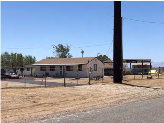
Detail view of Main House facade from 100th Street facing southeast
