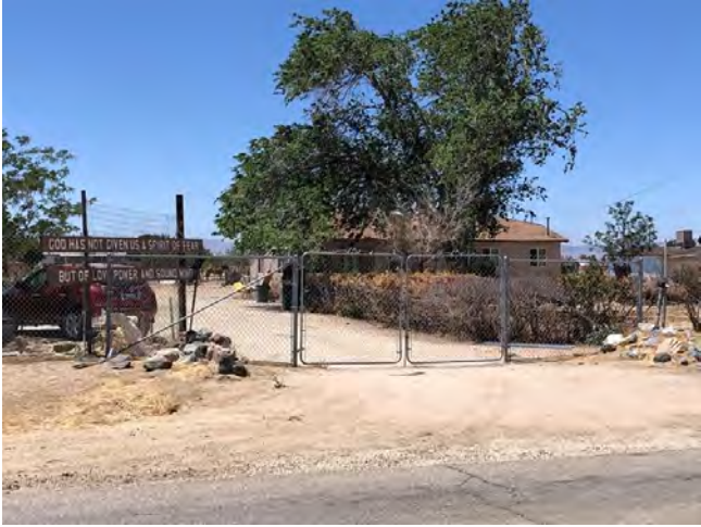
NE corner, showing east and north facades, facing southwest
