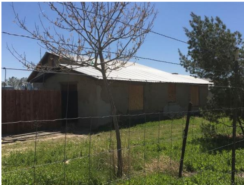
Photograph 8. Primary (west) and north elevations of Building H8, looking southeast
