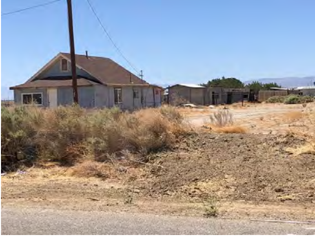
NW corner, showing west and north facades, facing southeast
