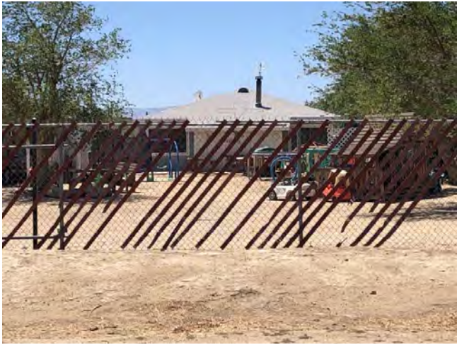
North elevation, view facing south from roadway
