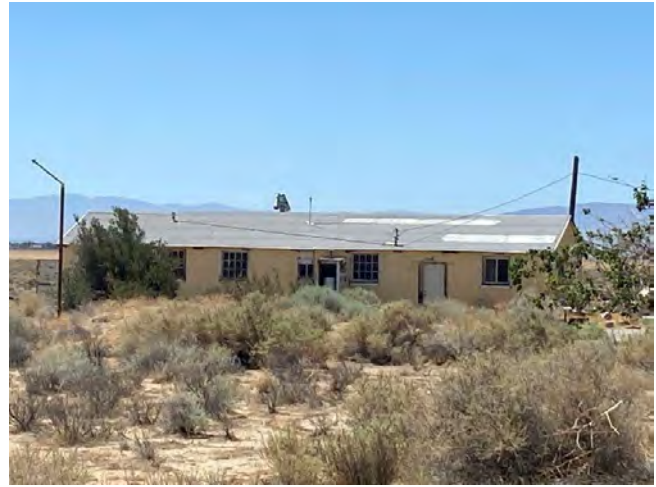
Secondary House north elevation, view facing south from Rosamond Blvd
