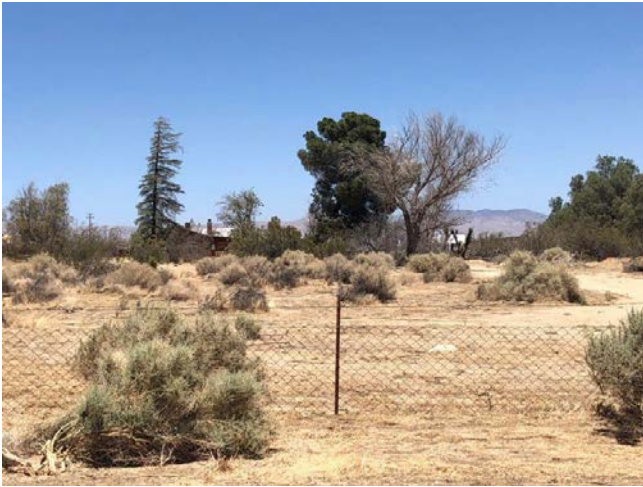
South elevation of the residence behind trees, facing north from roadway
