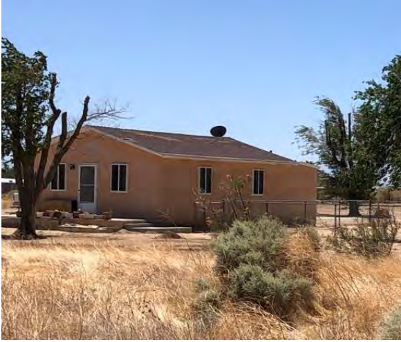
North and west elevations, facing southeast
