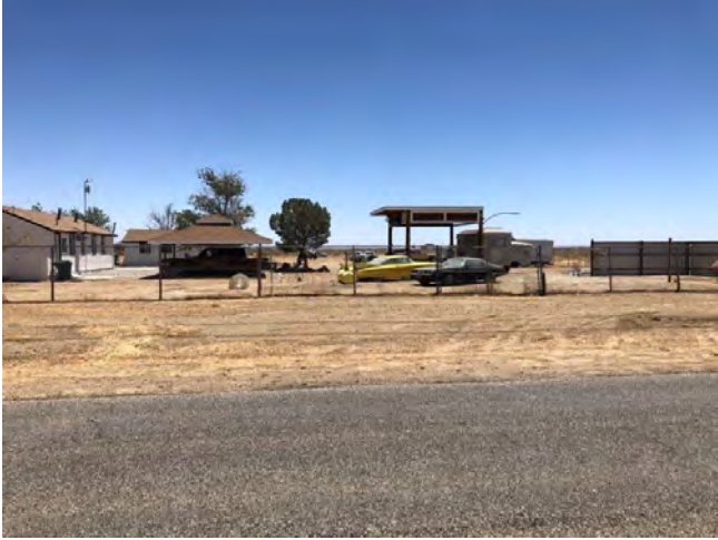
Rear elevation of Main House; view of Carport and Shelter from 100th Street facing east; west elevation of Detached Garage One
