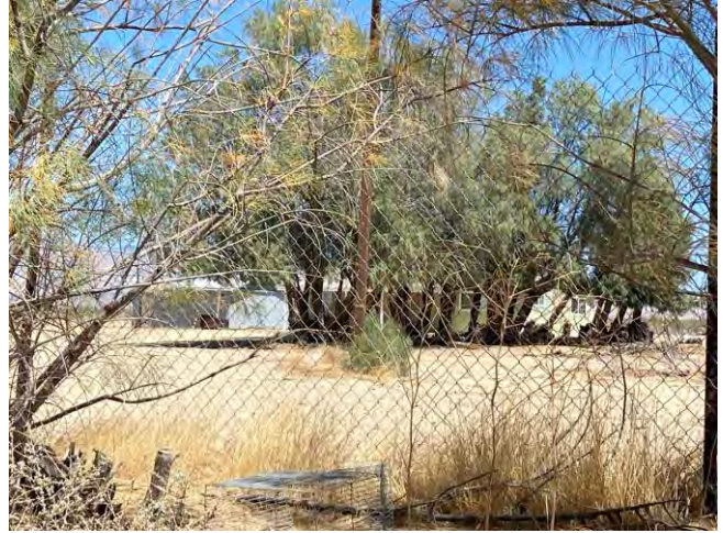
House 1 east elevation, facing northwest
