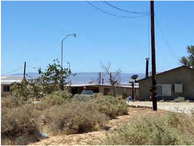
Outbuilding north elevation, view facing south from Rosamond Blvd
