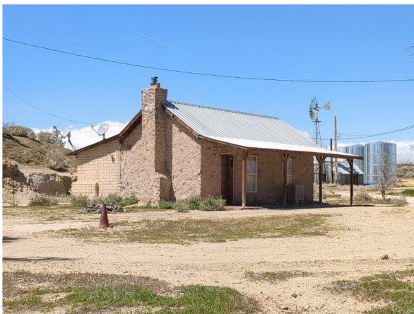
Photograph 13. Overview of Building H13 with Building A2 in the background, looking northwest
