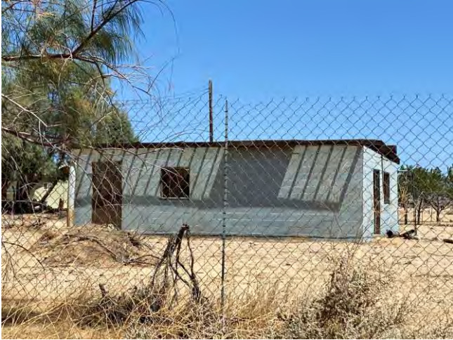
Outbuilding 2 south elevation, facing north
