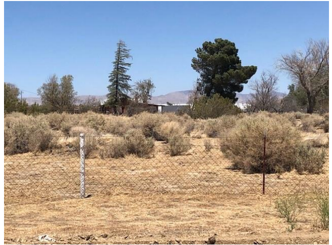
Additional view of south elevation of the residence, facing north from roadway
