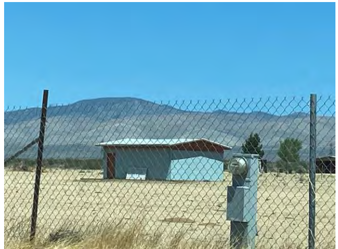
Outbuilding 1 south elevation, facing north
