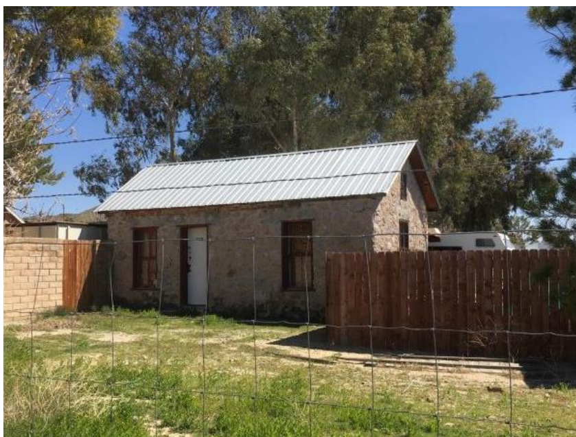
Photograph 9. Primary (west) and south elevations of Building H9, looking northeast
