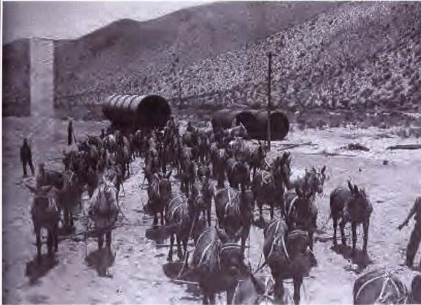
Photo 1, 52 Mule Team hauling pipe for the Jawbone Siphon
