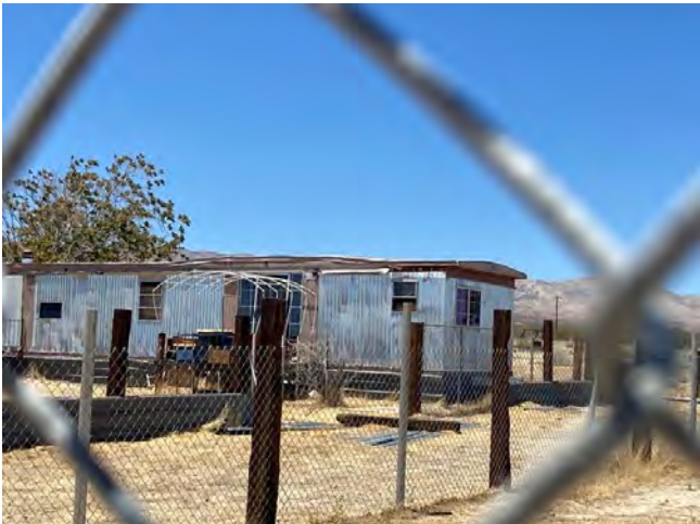
East manufactured home home, south elevation, view facing northeast
