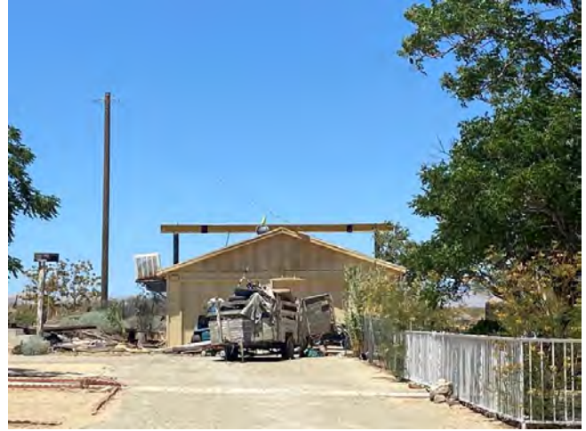
Garage, south elevation, view facing north
