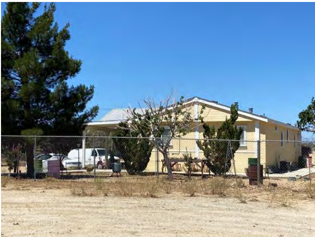
House 2 east elevation, facing west
