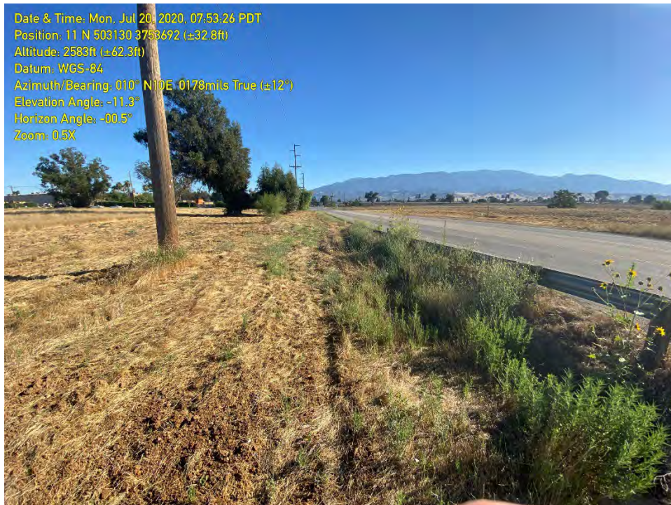
PHOTOGRAPH 4: No roadside drainage was present, or evidence thereof, indicating all flow for Feature A originated from road runoff.
