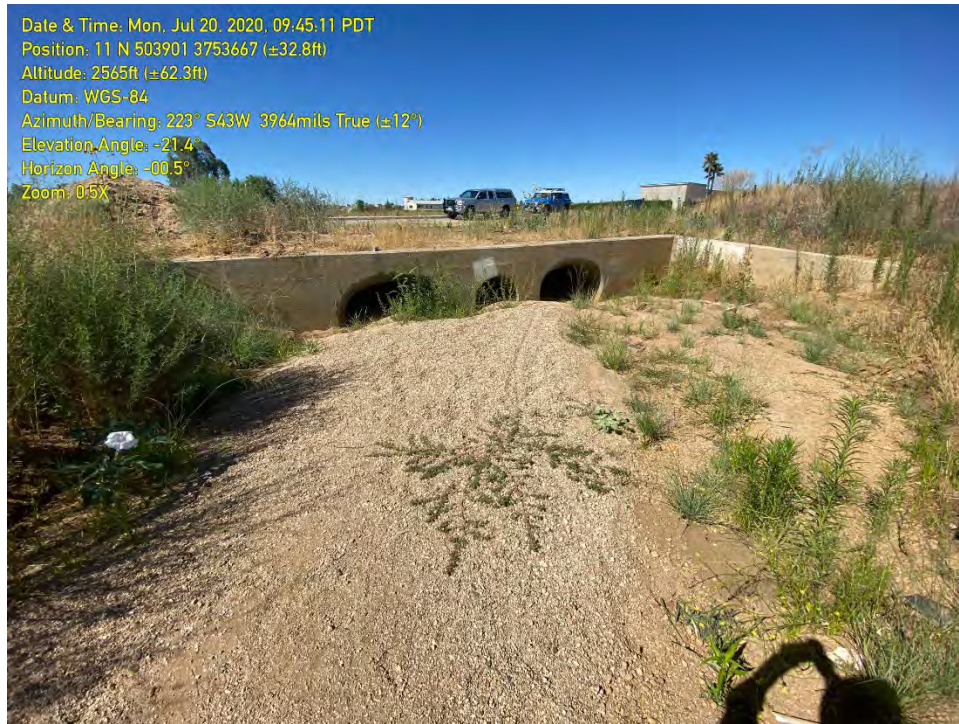
PHOTOGRAPH 7: The culvert at 2 nd Street from the upstream end of Feature C (Potrero Creek).
