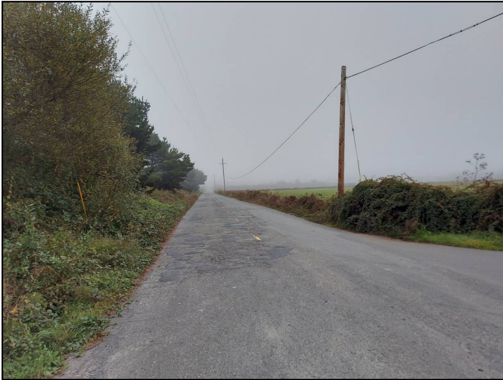
11 : View down Foster Avenue, facing southeast.
