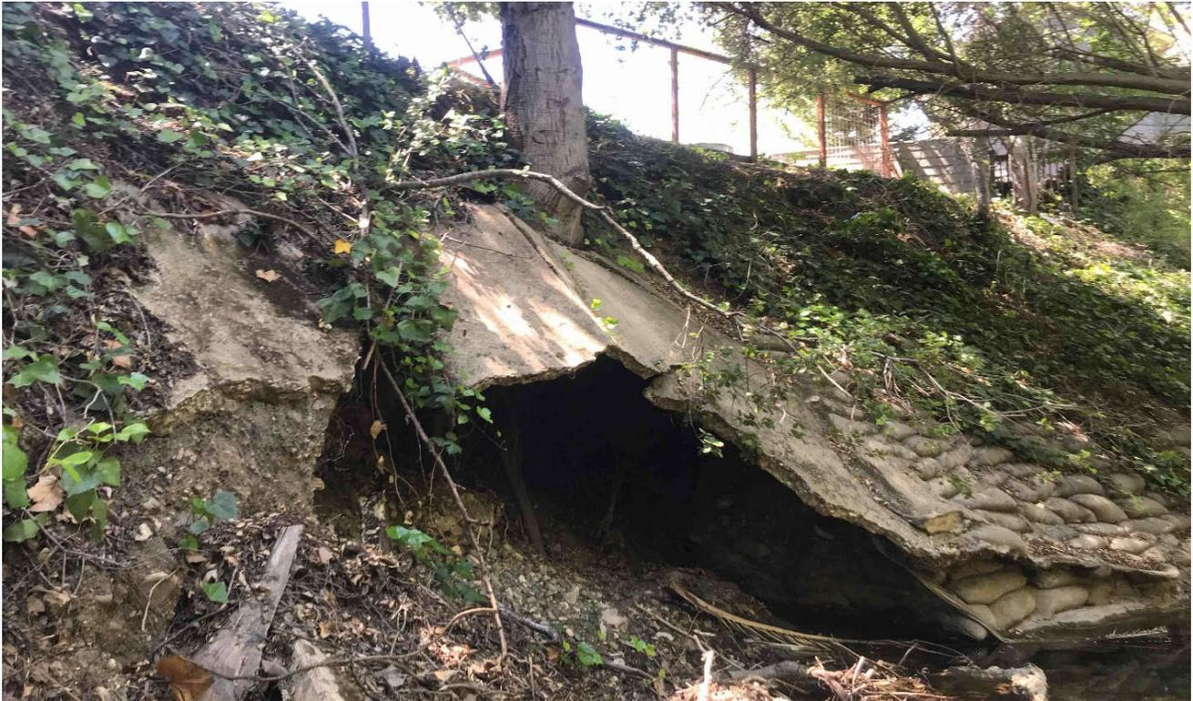
**Photograph 1.** View of the south bank of San Luis Obispo Creek where the concrete infrastructure has been undercut and eroded by water flow (facing south, May 3, 2022).
