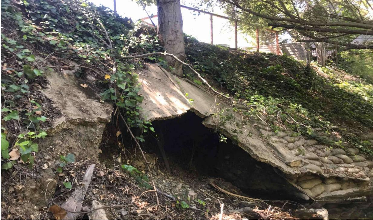
**Photograph 5.** A closer look at the south bank of San Luis Obispo Creek where the concrete infrastructure has been undercut and eroded by water flow (facing south, May 3, 2022).
