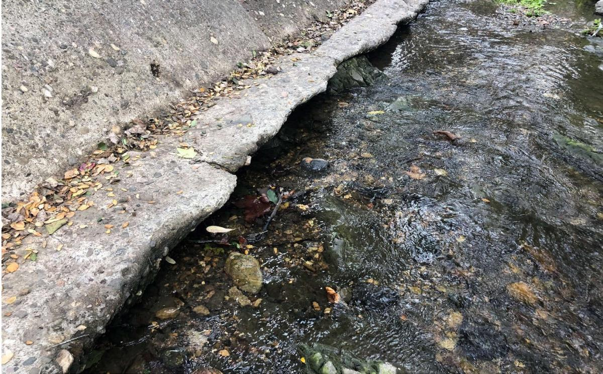
**Photograph 5.** View of the eroded base of the existing slope protection infrastructure, facing southwest (downstream).
