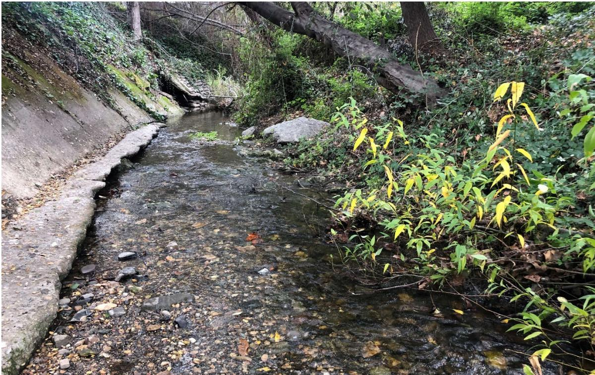
**Photograph 4.** View of San Luis Obispo Creek and the existing concrete slope protection infrastructure immediately downstream of the Johnson Avenue bridge, facing southwest (downstream).
