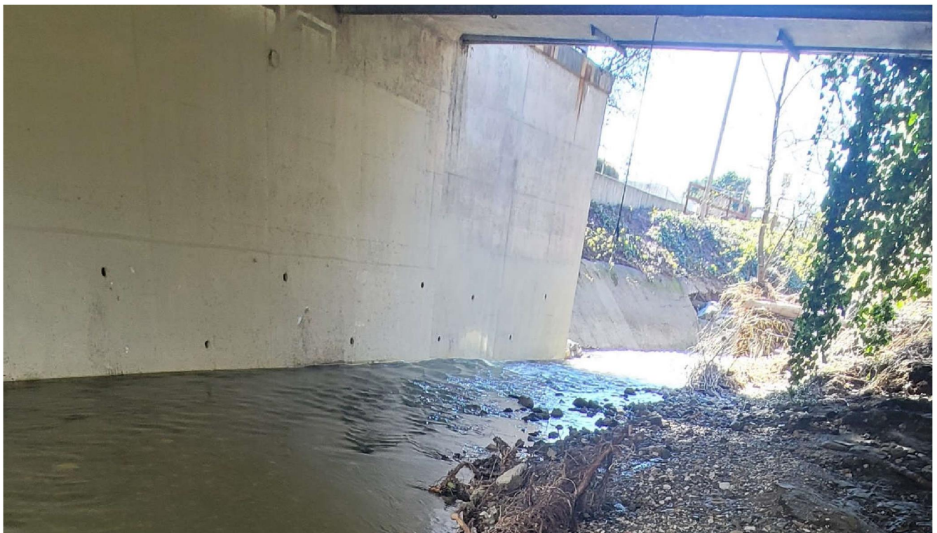
Photograph 4. The natural bottom culvert underneath Johnson Avenue following (facing northeast, January 26, 2023).
