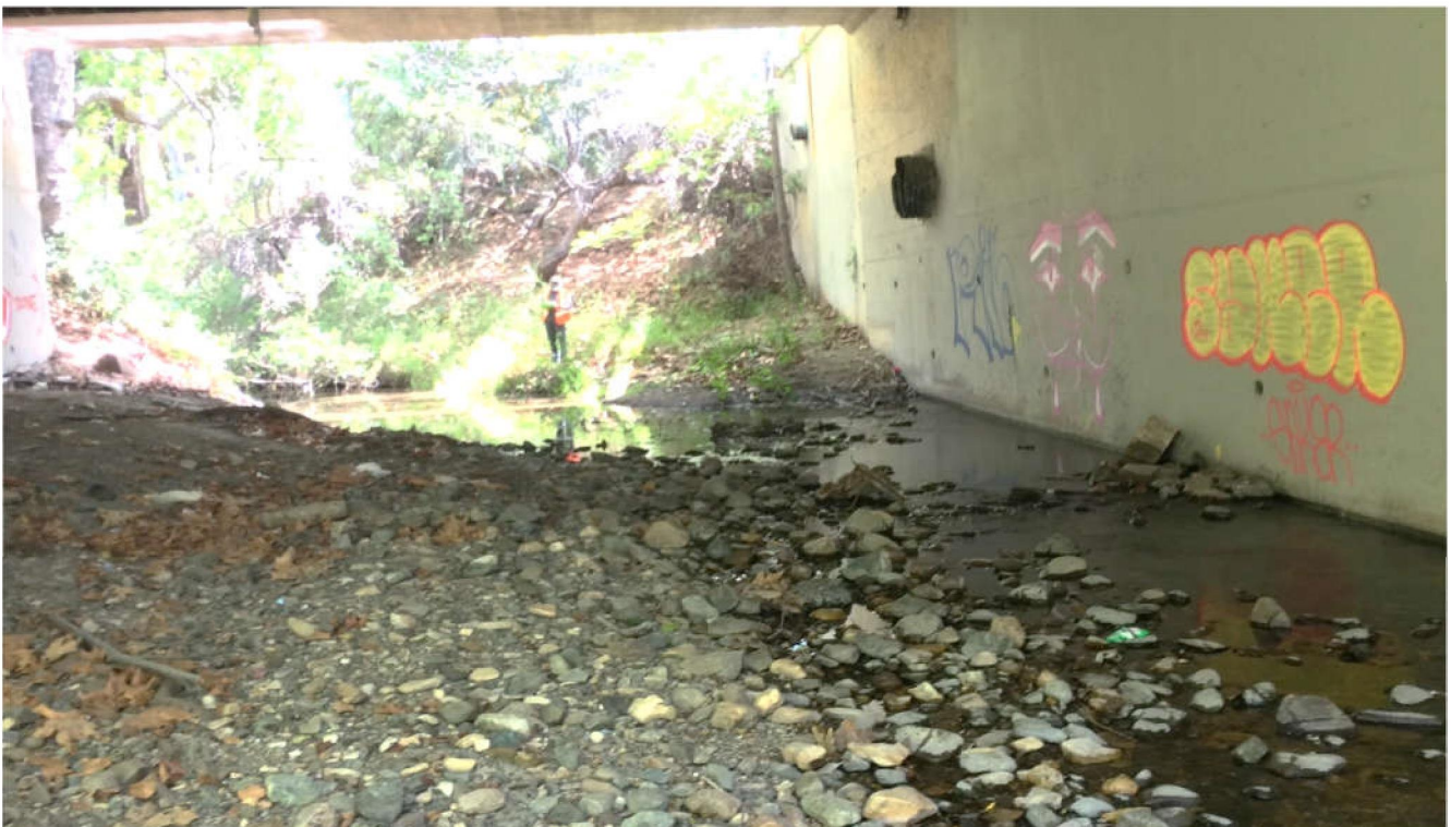
Photograph 2. The natural bottom culvert underneath Johnson Avenue (facing northeast, May 3, 2022).
