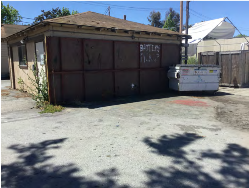
Photograph 9: View of northern side of industrial office building, "Battery Pickup" area, and solid waste dumpster; located in the south-central portion of the Subject Property. View looks towards the southwest.
