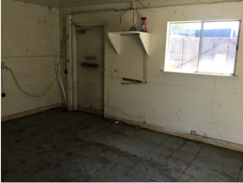
Photograph 5: Interior of industrial office building in south-central portion of Subject Property.
