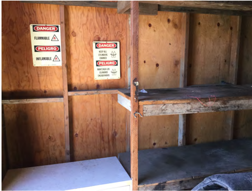
Photograph 7: Shelves inside of wooden storage shed with signs indicating past storage of cylinders and flammables.
