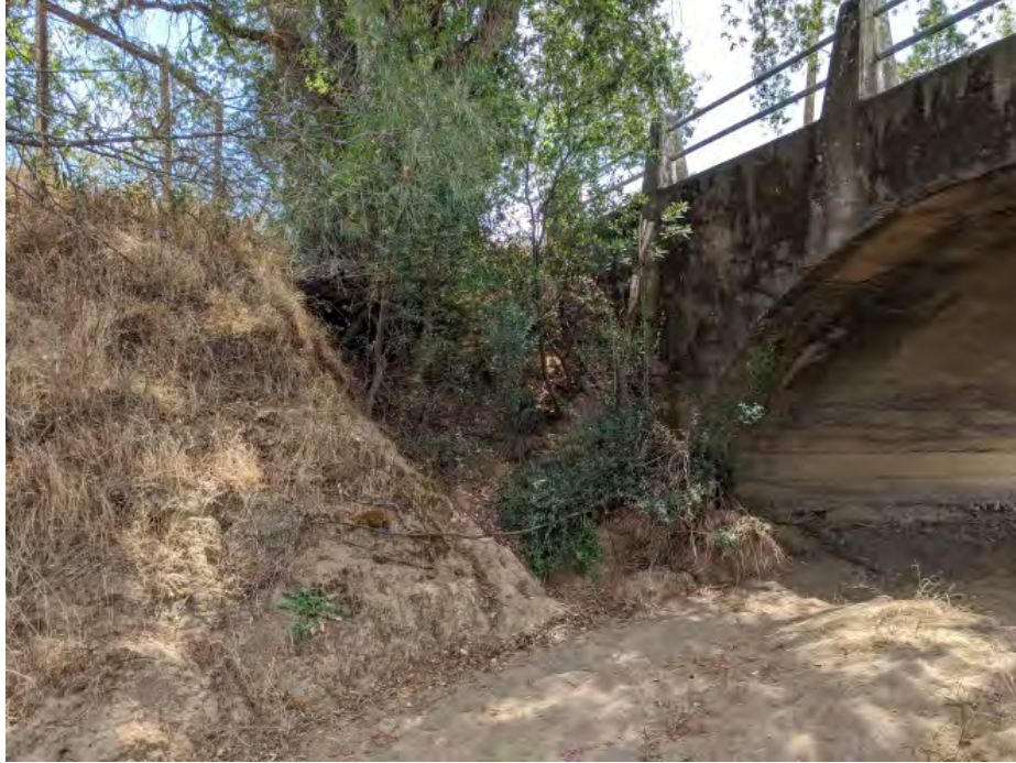
Overview of Hamilton Creek and current bridge, looking southeast.
