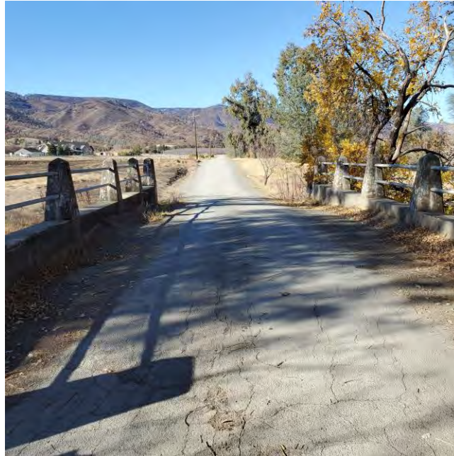
Figure 6. Project overview, viewing northwest
