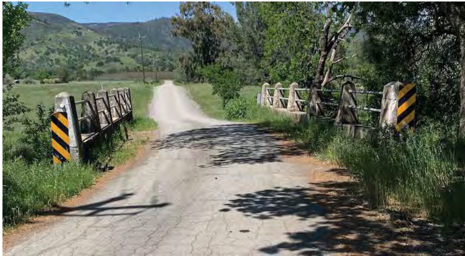
Photo 2. View of bridge toward the northwest.
