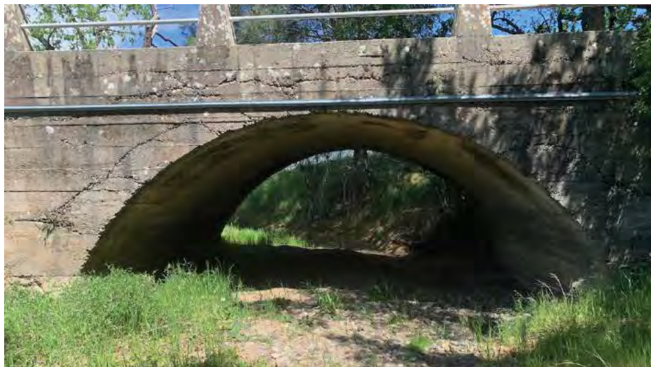
Photo 3. View of bridge toward the northeast.
