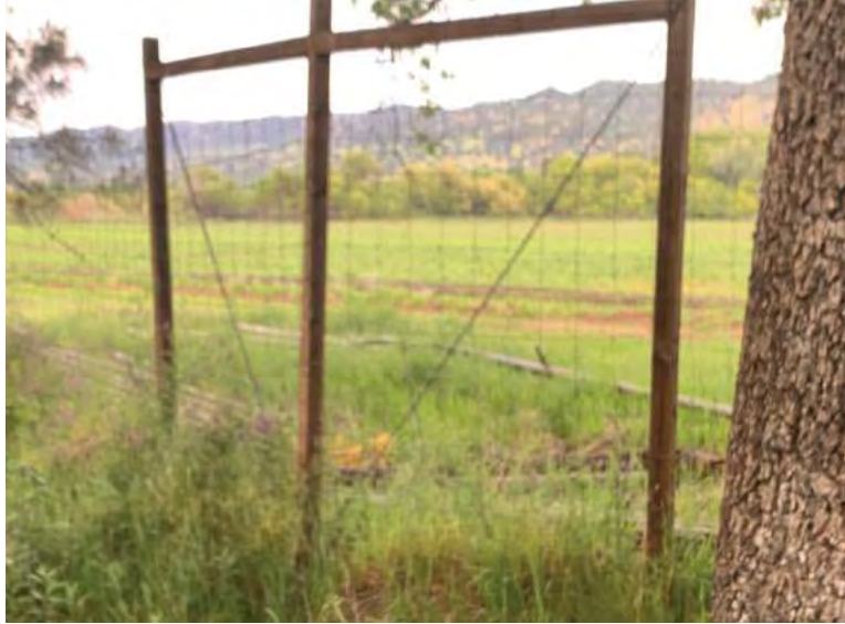
Photo 6. APN 060-090-002; treated wood fencing.
