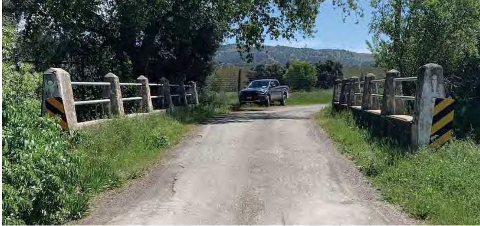
Photo 1. View of bridge toward the southeast.
