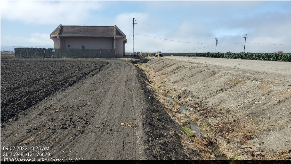
Photograph 2. The roadside drainage east of Watsonville Road and existing M1W pump station, facing south. September 2, 2022.
