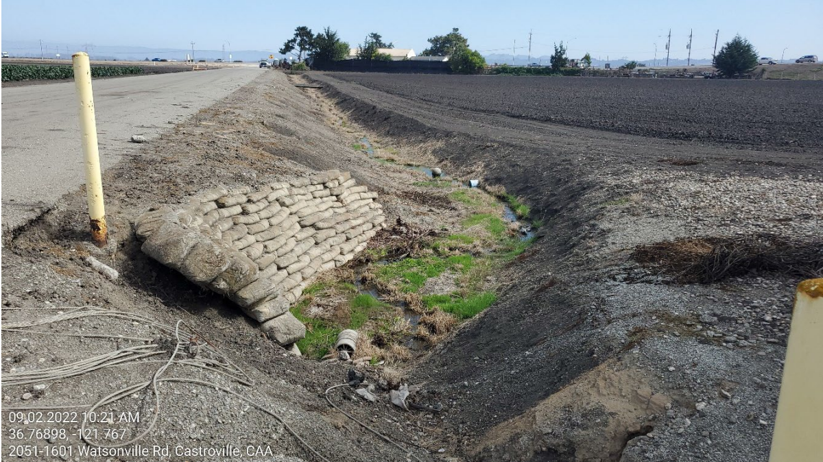
Photograph 1. The roadside drainage east of Watsonville Road, facing north. September 2, 2022.
